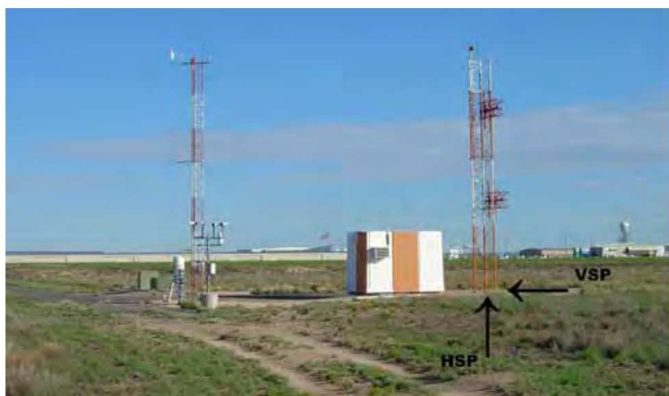
Figure C-6. Typical glideslope installation.
