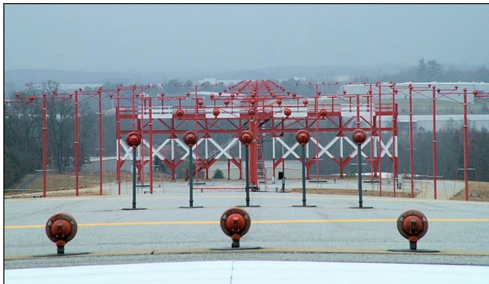
Standard ALS installation. Note electrical metallic tubing (EMT) with frangible couplings installed on light stations that are less than 6 feet high.
