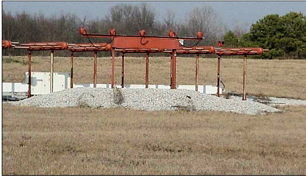
Figure B-2. Unacceptable Grading Surrounding NAVAIDs
