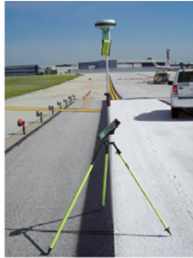
Correctly placed survey equipment
