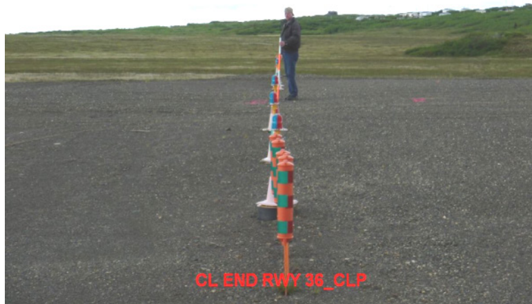
Figure 2-9. Illustrates the Use of Day Markers to Define the End of a Runway
