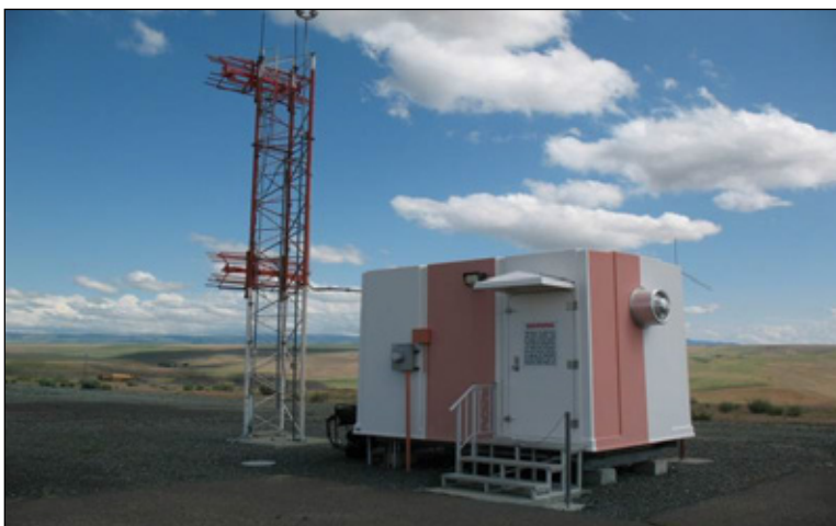
Figure 6-24. GS antenna and equipment shelter
