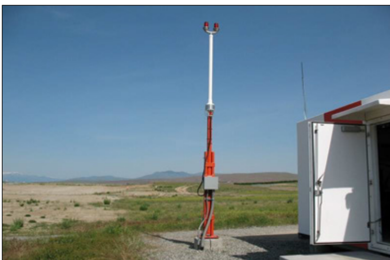
Figure 6-25. Distance Measuring Equipment (DME) antenna
