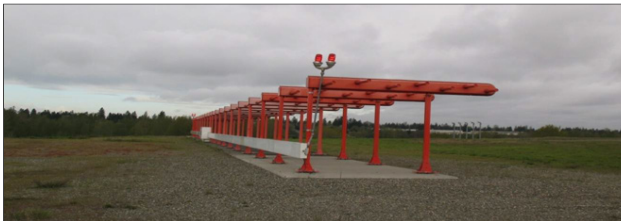
Figure 6-22. LOC 14-antenna array
