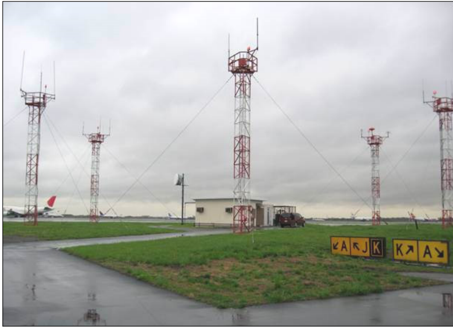
Figure 6-4. Remote Transmitter/Receiver (RTR) communication facility
