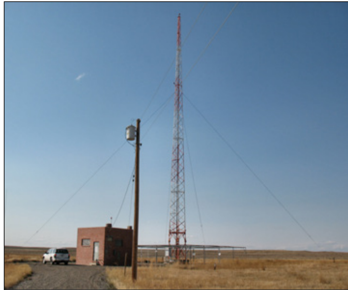
Figure 6-31. Non-Directional Beacon (NDB) facility
