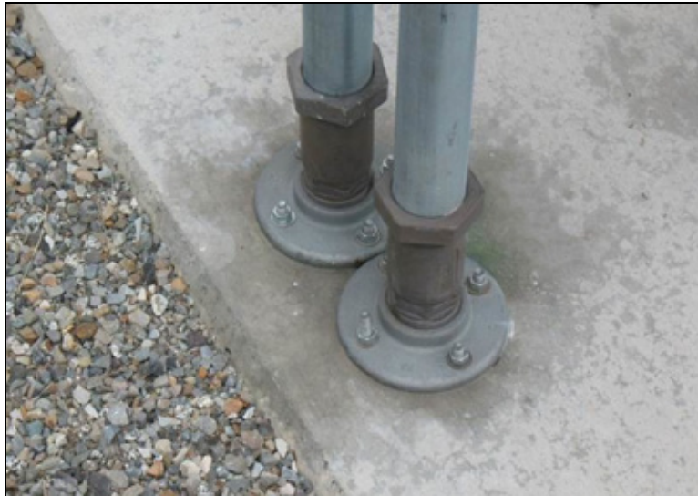
Figure 6-2. Two frangible connections
