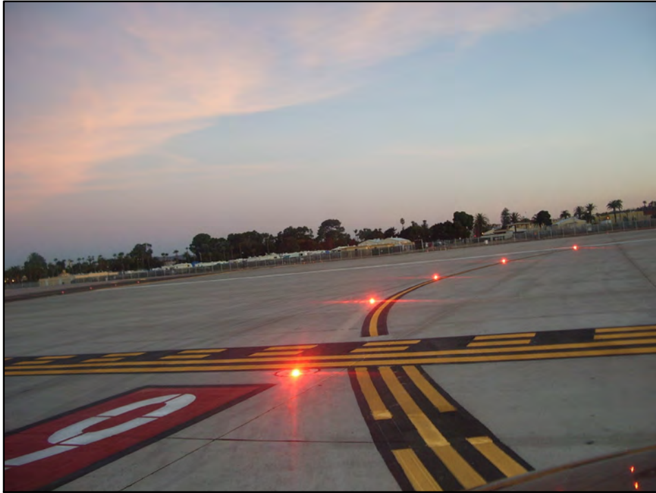
FIG 2-1-10 Runway Entrance Lights
