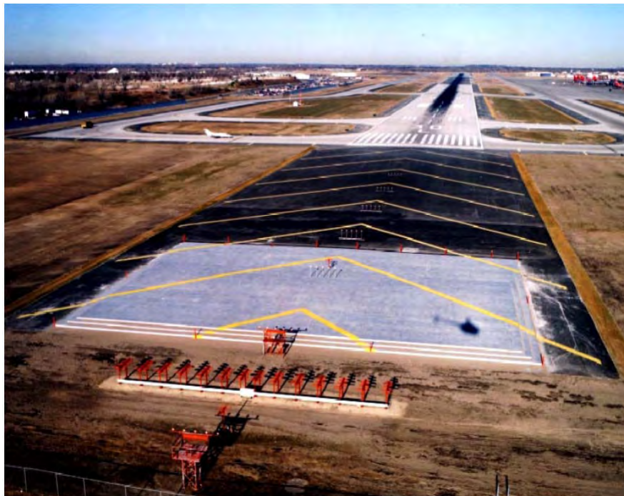
FIG AD 1.1-54 Engineered Materials Arresting System (EMAS)
