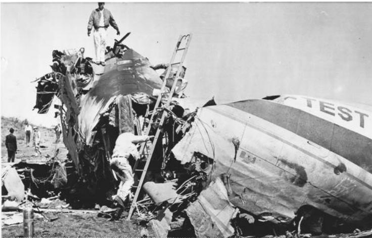
Twelve of the 16 dummies remained seat-belted in their seats as the plane came to rest on its left side. Surprised by the amount of damage to the plane, researchers were even more astonished that most passengers would have survived the crash. Using the data culled from the crash, researchers hoped to help strengthen items such as
