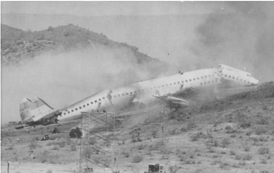
In the second test, engineers remotely sent the Constellation down a 4,000-foot runway where it hit a series of strategically placed barriers at 115 miles per hour. Both wings separated from the aircraft and the fuselage broke in two
