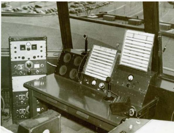
When the LaGuardia Tower became a federal facility in 1943, the CAA installed a radio desk and flight strip assembly, which probably made it the first approach control set up in the eastern U.S.
