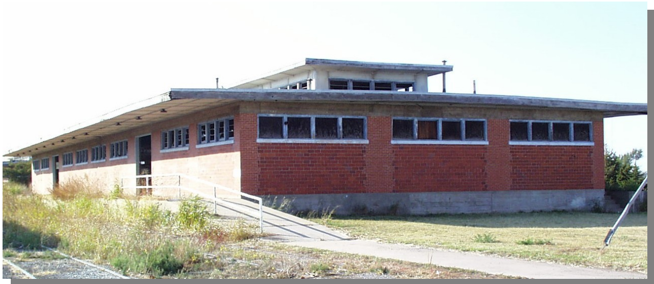
Exhibit 3-29. Building 208 in Warehouse Area
