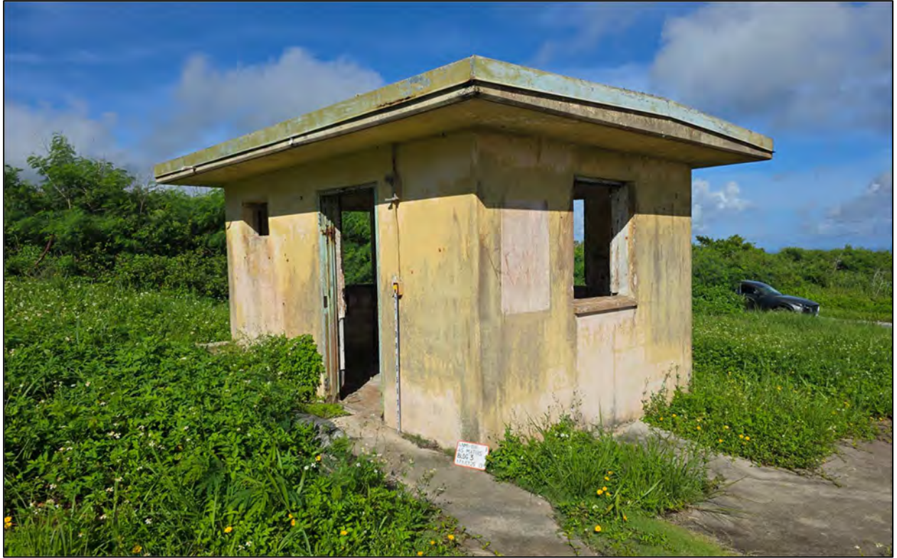
Figure 39: View southwest of Building 3 - guard house.
