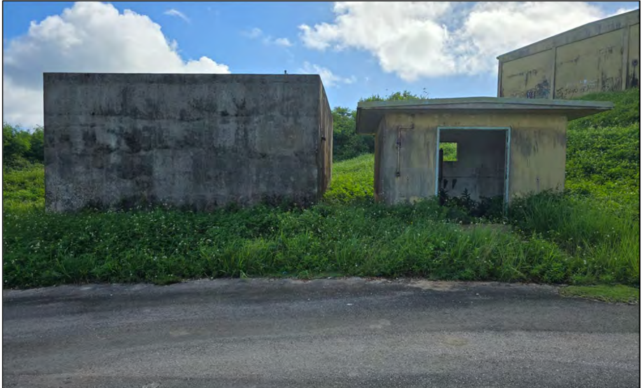
Figure 40: View north of Building 4 and water tank.
