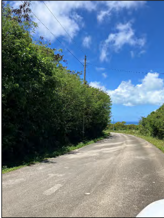
Picture 5: Existing single-phase electrical line distribution (ELD) wooden poles along Pale Arnold Road.
