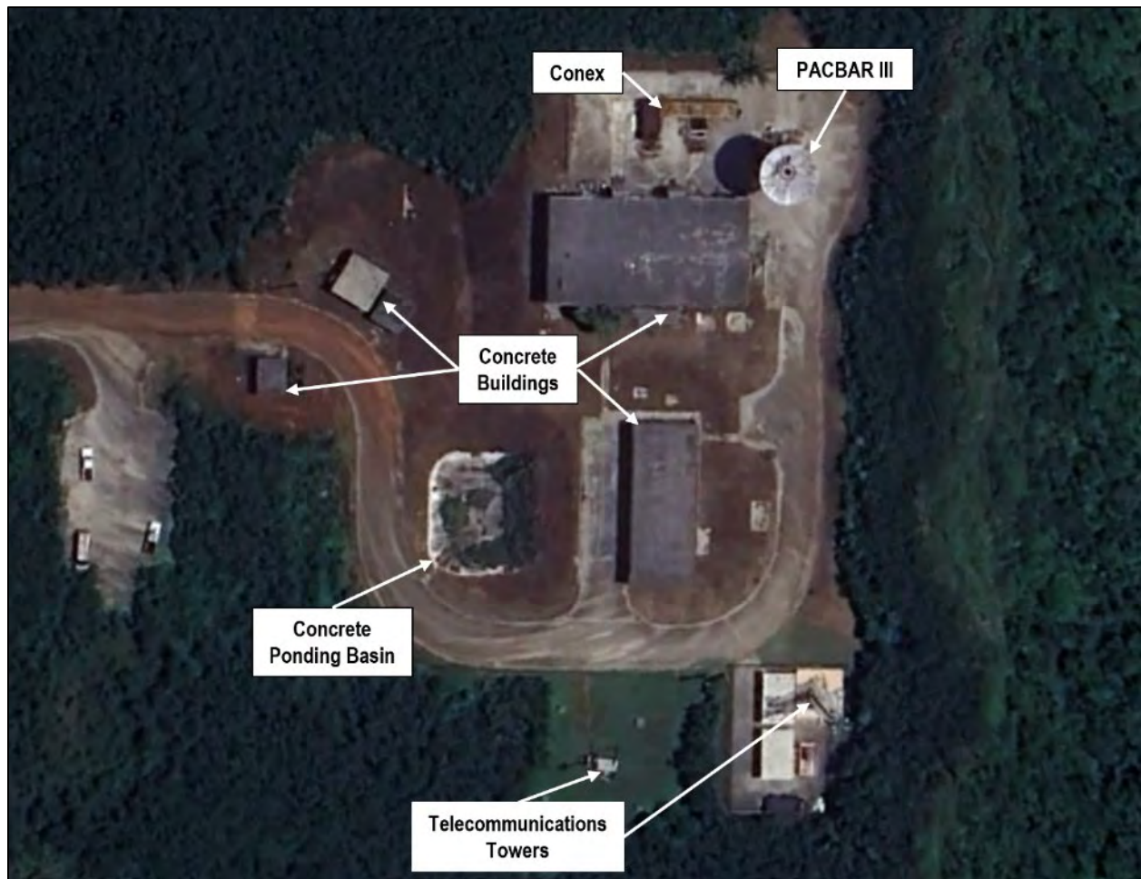
Figure 3-6 Aerial view of the Mount Petosukara summit showing the existing radar installation site and remaining infrastructure associated with the former PACBAR III radar facility. The proposed ARSR facility would be constructed within this previously developed footprint. Source: Google Earth Imagery accessed March 2026.
