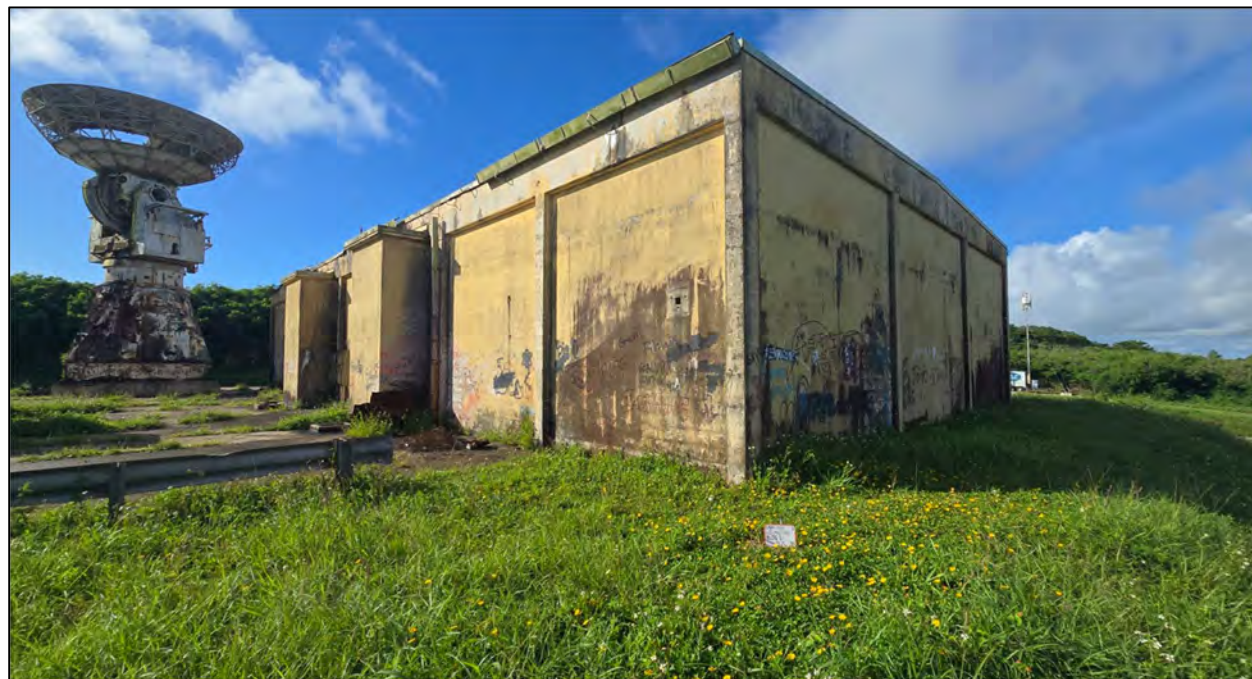
Figure 32: View southeast of Building 1 – operations – and radar.
