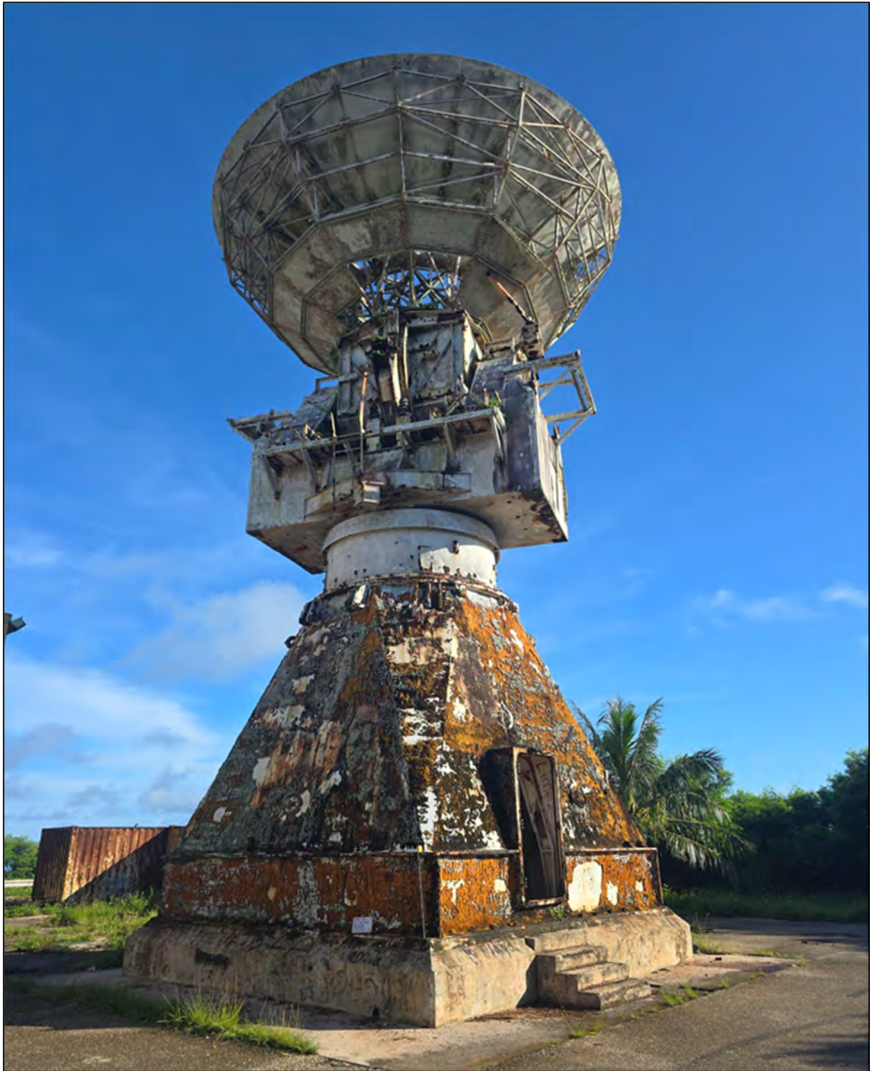
Figure 27: View north of radar structure and C-band dish.
