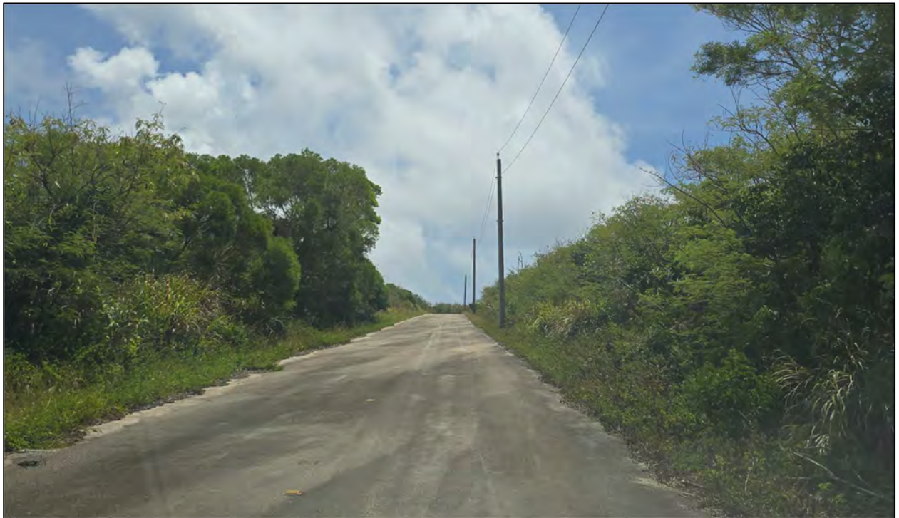
Figure 13: View east from east portion of straightaway of Area 4.
