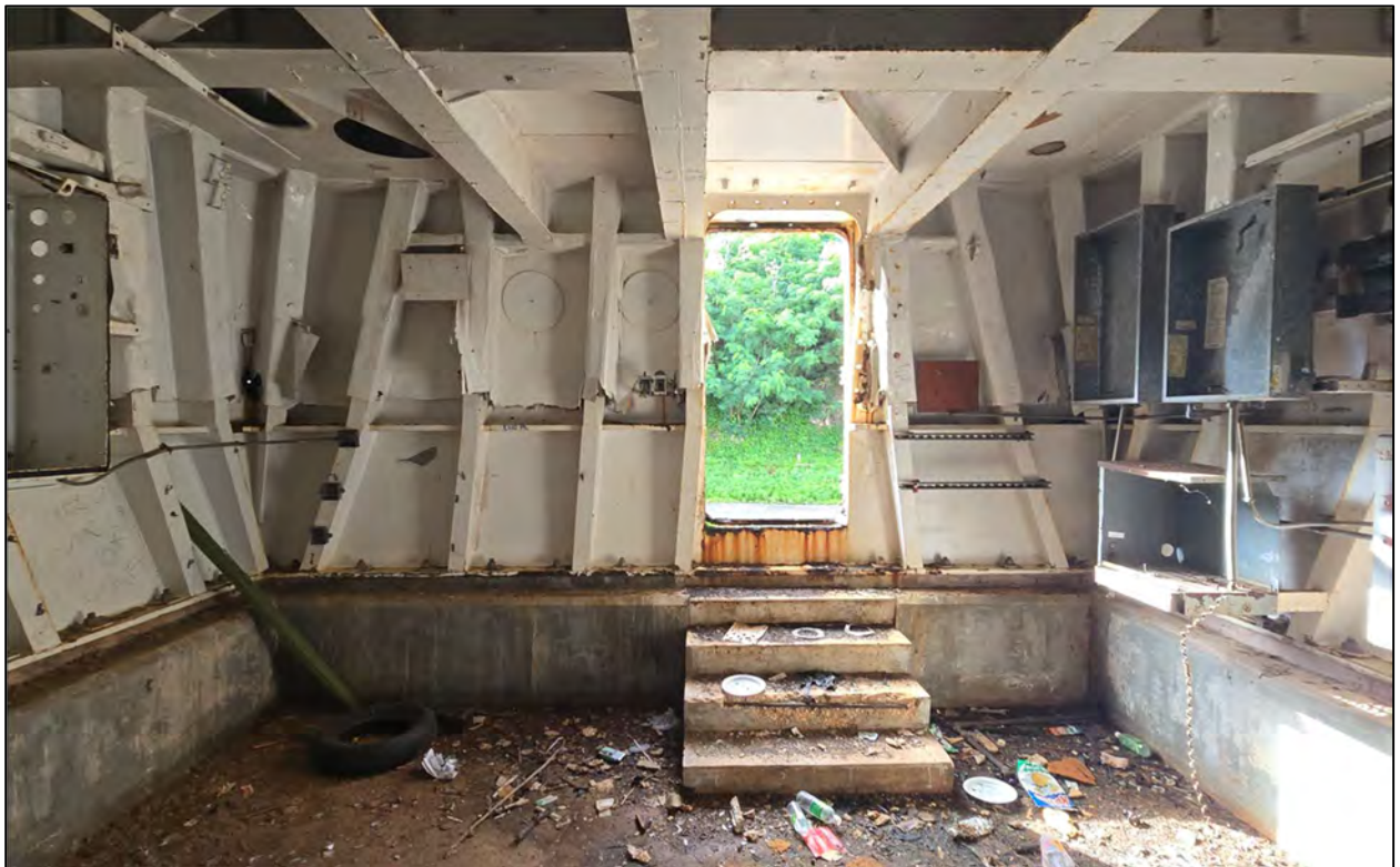
Figure 30: View of interior of radar structure.
