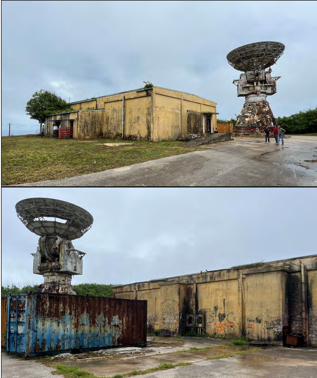
Figure 3 Existing PACBAR III Facility atop Mount Petosukara. The facility is no longer operational and would be removed as part of the Proposed Action.
