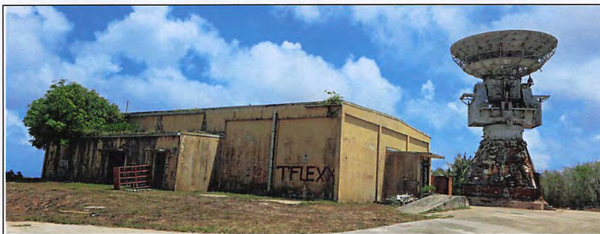
Figure 22: View north of the PACBAR III radar and operations building.
