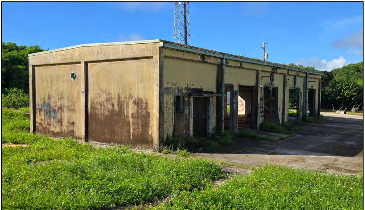
Figure 36: View southeast of Building 2.
