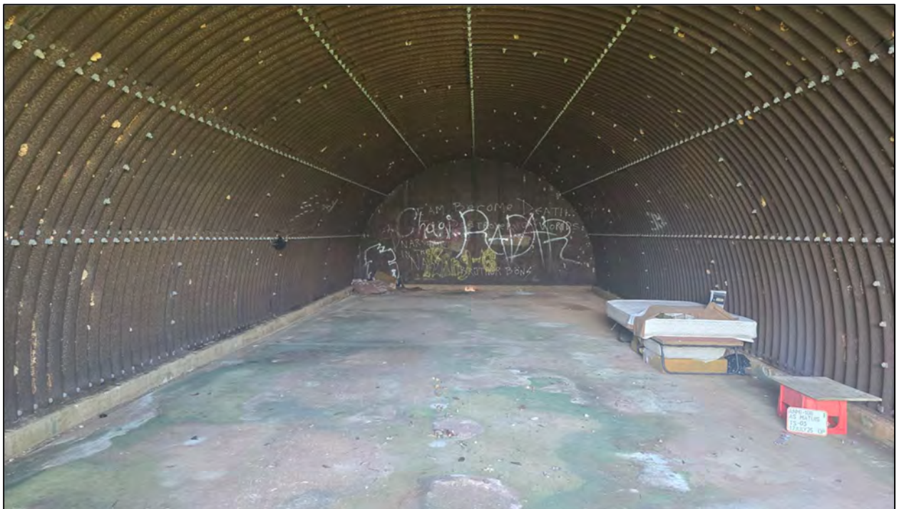
Figure 24: View of interior of TS-3.
