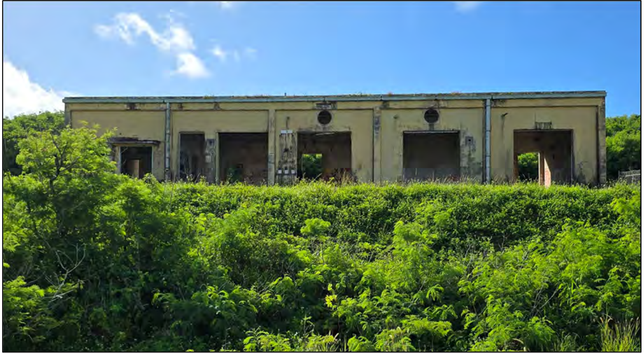
Figure 35: View east of Building 2 - maintenance.
