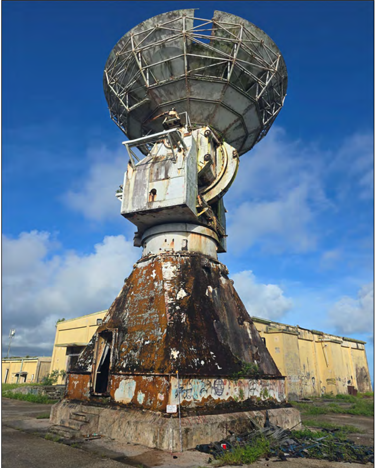
Figure 28: View west of radar structure.
