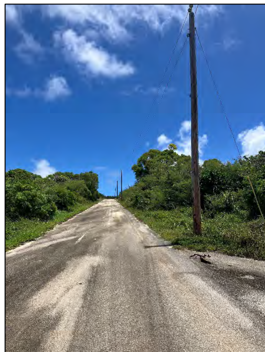
Picture 4: Existing single-phase electrical line distribution (ELD) wooden poles along Pale Arnold Road d.
