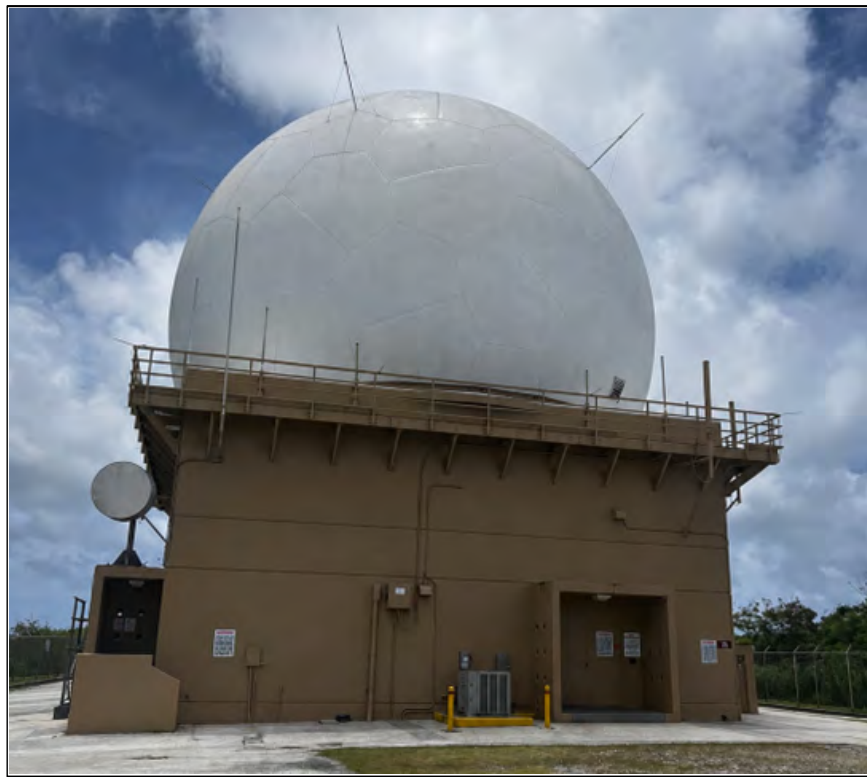
Figure 2-5 Representative FAA Air Route Surveillance Radar (ARSR) facility showing the radome mounted directly on the roof of the radar operations building.
