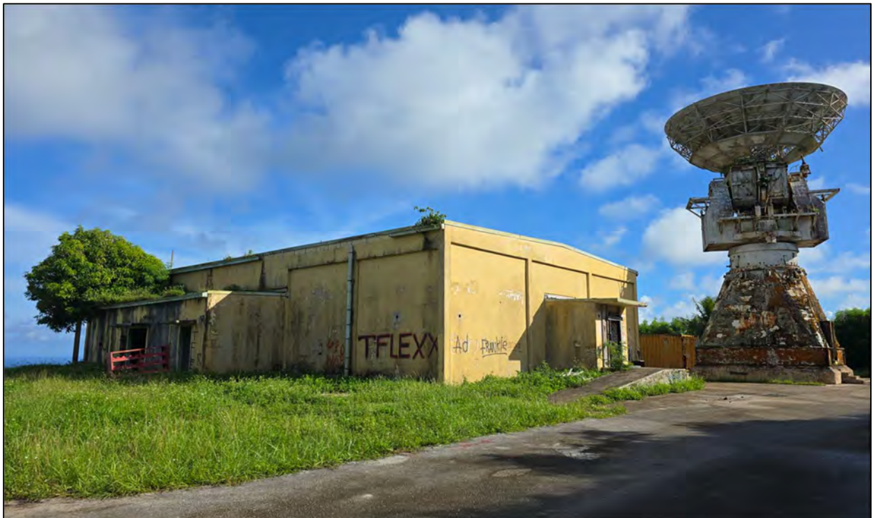
Figure 34: View northwest of Building 1 and radar.
