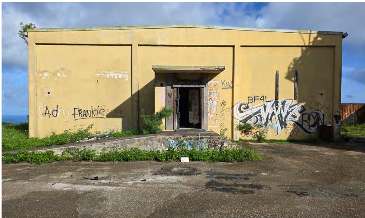
Figure 31: View west of front of Building 1 - operations.
