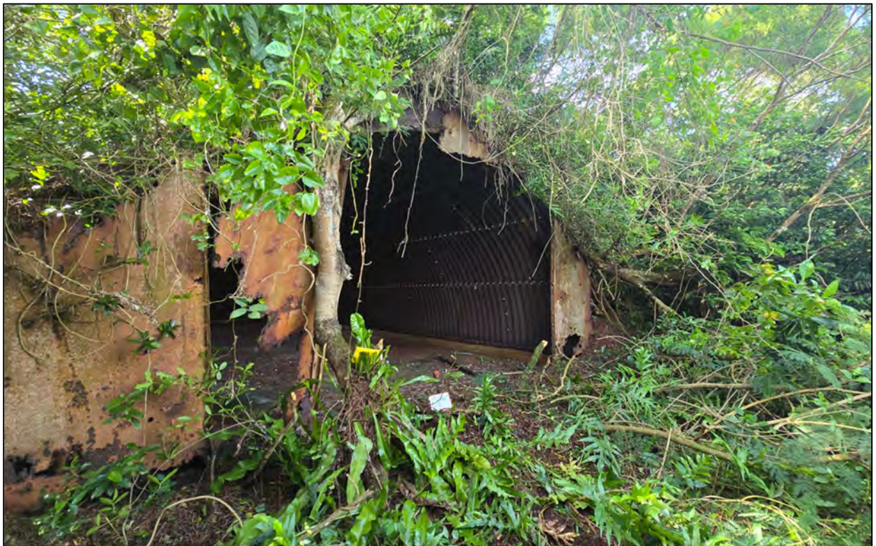
Figure 22: View south of front of TS-2.
