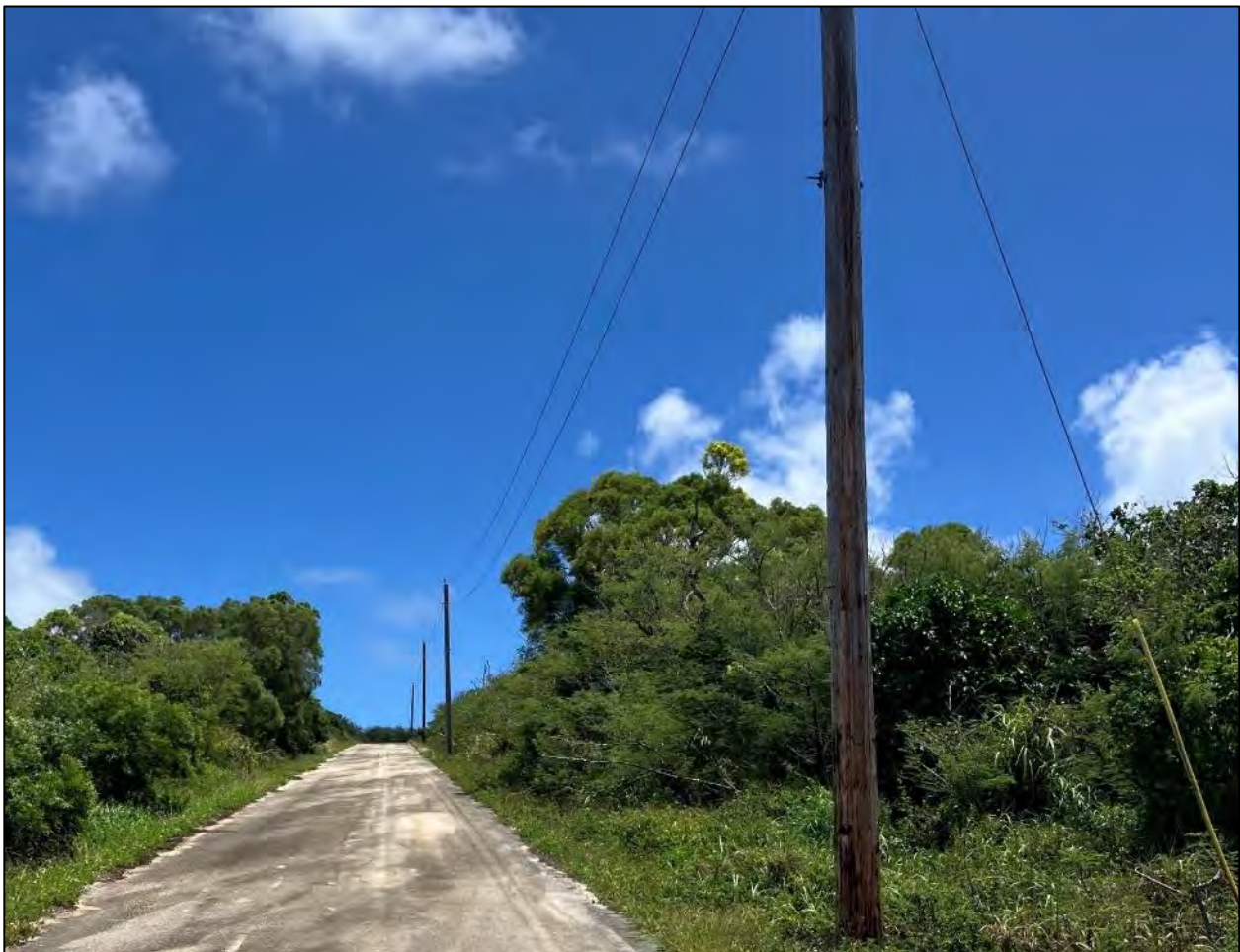
Figure 2-4 Existing single-phase electrical distribution line (ELD) along the radar access road.
