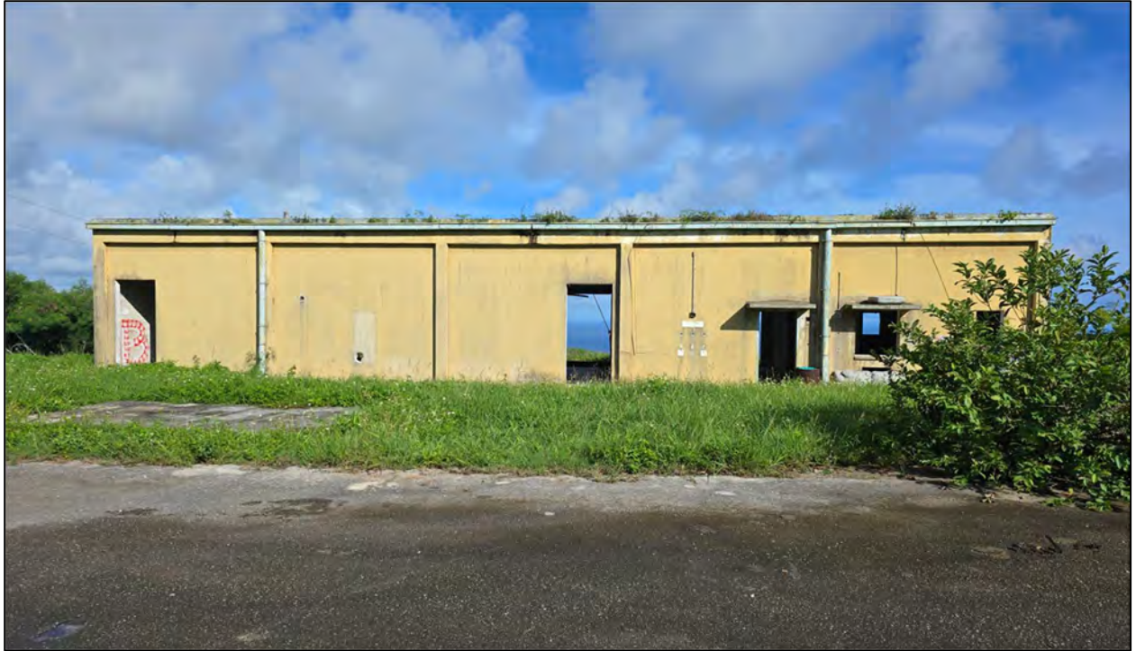
Figure 37: View west of Building 2.
