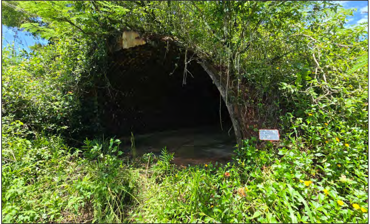
Figure 23: View northeast of front of TS-3.
