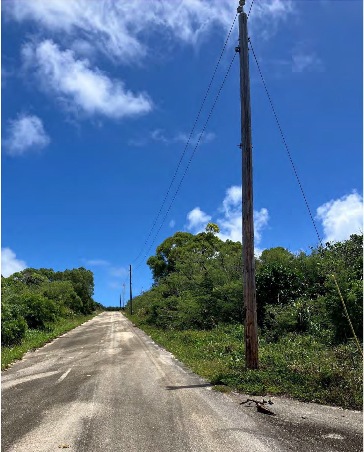
Figure 4 Existing single-phase ELD along the radar access road. The Proposed Action would upgrade this system to three-phase power with concrete poles to support operation of the new ARSR facility.
