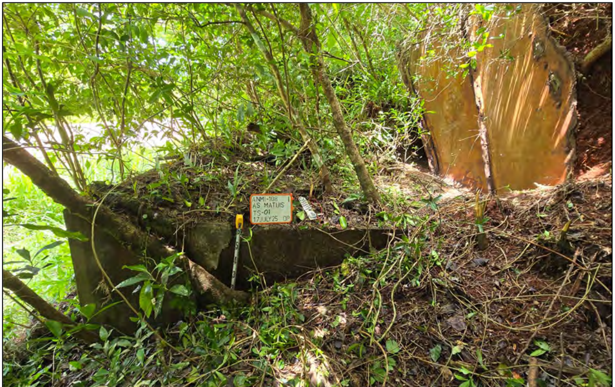
Figure 20: View north of side of loading area at TS-1.
