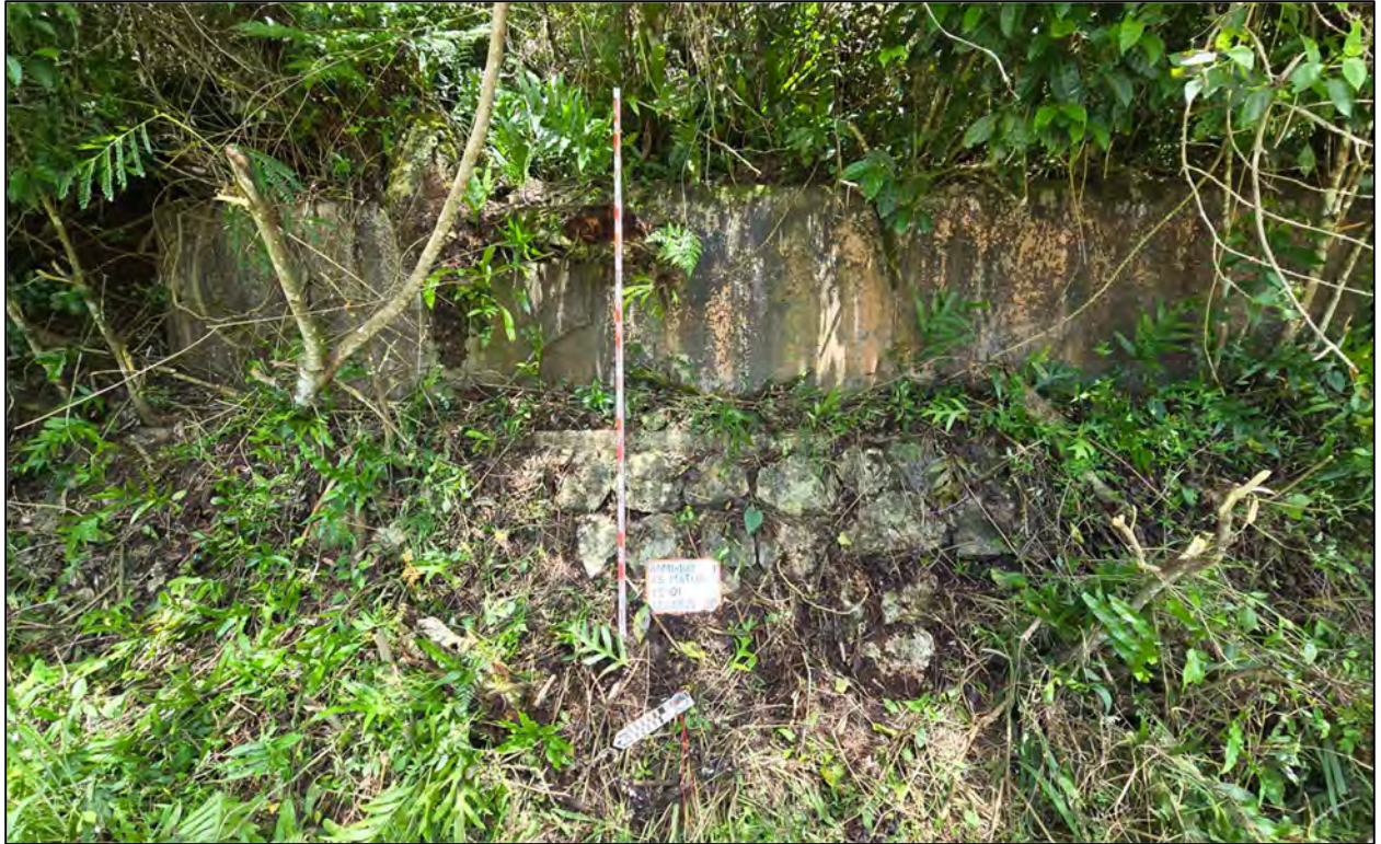
Figure 19: View southeast of stone facing below TS-1 loading area.
