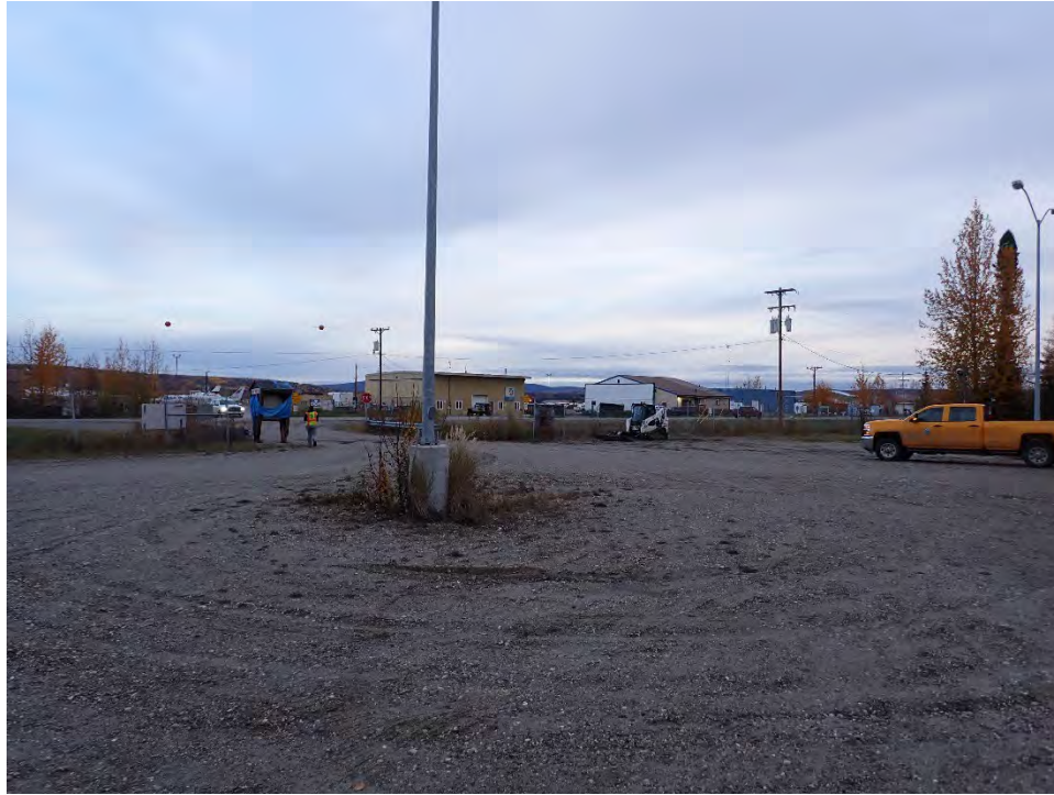
Photograph 11: Previously cleared area in southwest portion of new ATCT/TRACON site (facing northwest).
