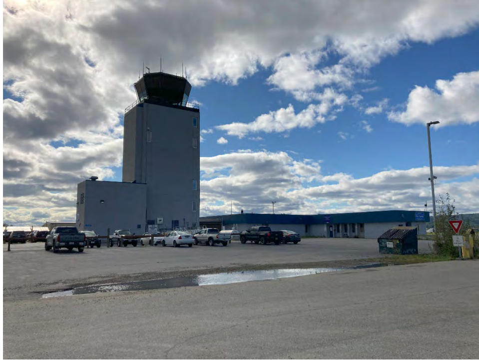
Photograph 13: Existing ATCT/TRACON (facing southwest).
