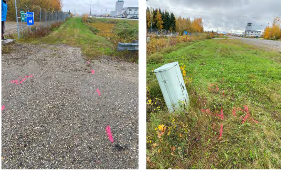
Photograph 1: Utility ROW and drainage ditch along University Avenue South, Lease Lot 6A (facing southwest).
