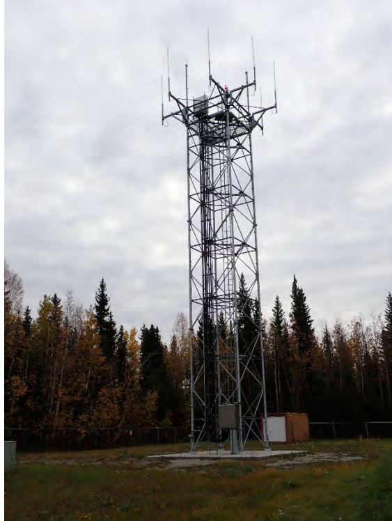
Photograph 3: Remote Transmitter/Receiver (RTR) building at northeast end of FAI (facing south-southwest).
