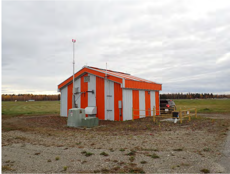
Photograph 1: Communications building (foreground) and FAI airfield (background; facing north-northeast).
