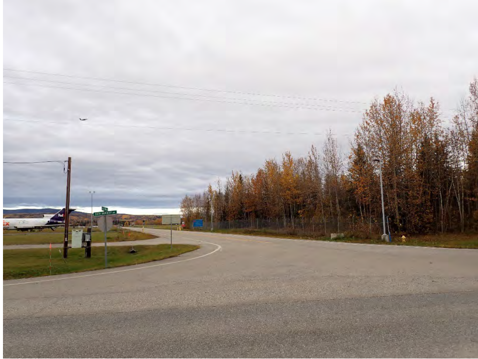
Photograph 5: Intersection of Float Pond Road and University Avenue South (facing northwest).
