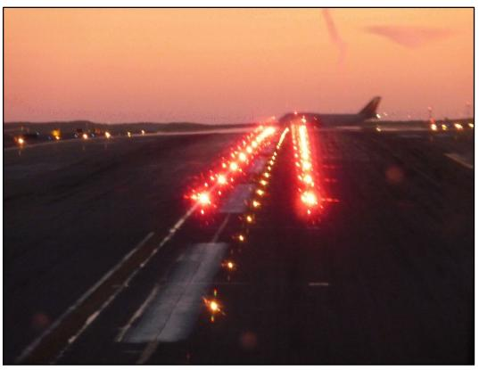
FIG 2-1-12 Taxiway Lead-On Light Configuration
