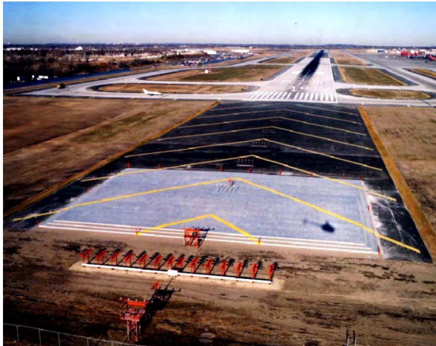
FIG AD 1.1-56 Engineered Materials Arresting System (EMAS)
