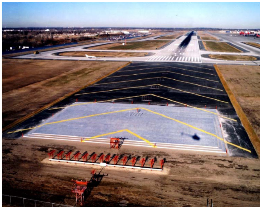
FIG AD 1.1-54 Engineered Materials Arresting System (EMAS)
