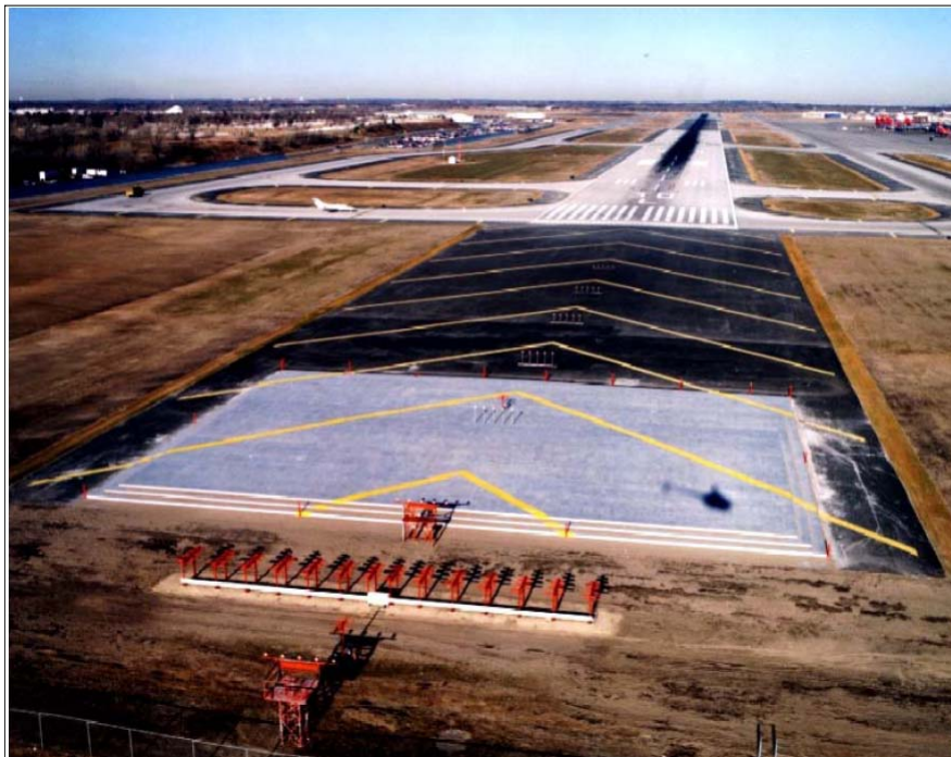
FIG 2-3-42 Engineered Materials Arresting System (EMAS)
