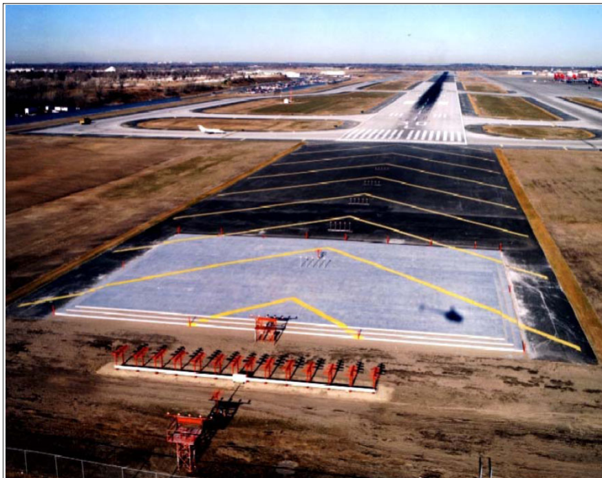
FIG 2-3-42 Engineered Materials Arresting System (EMAS)
