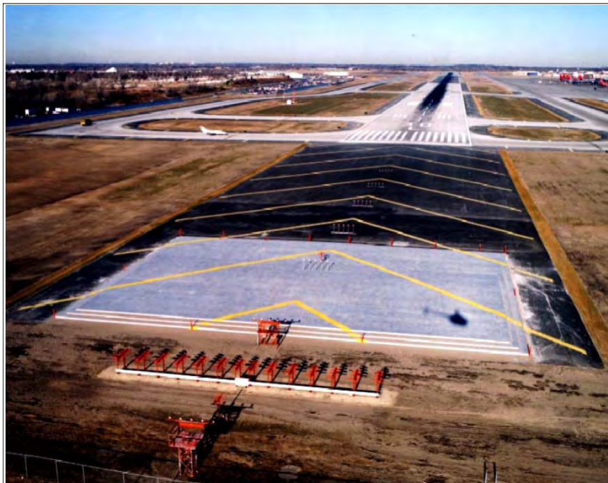
FIG 2-3-42 Engineered Materials Arresting System (EMAS)
