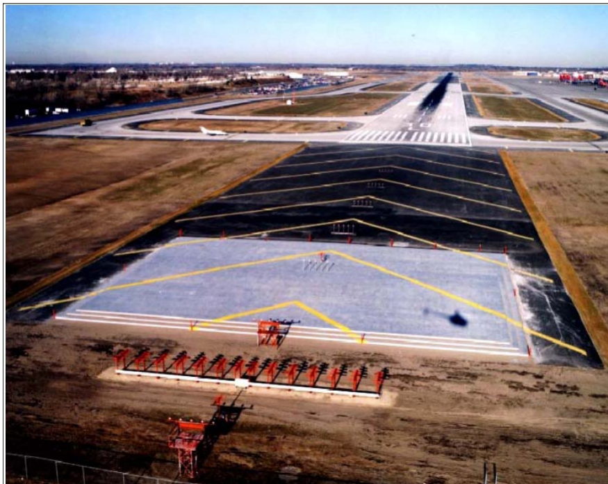
FIG 2-3-42 Engineered Materials Arresting System (EMAS)
