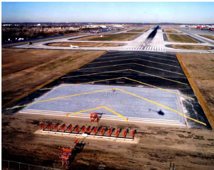
FIG AD 1.1-54 Engineered Materials Arresting System (EMAS)
