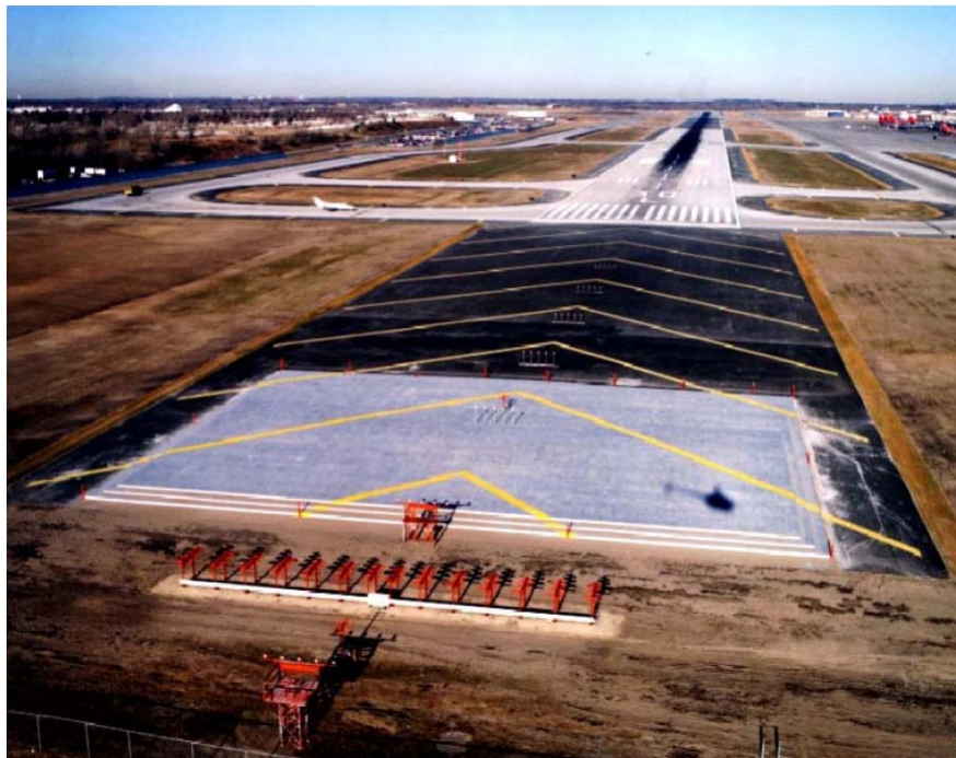
FIG AD 1.1-56 Engineered Materials Arresting System (EMAS)
