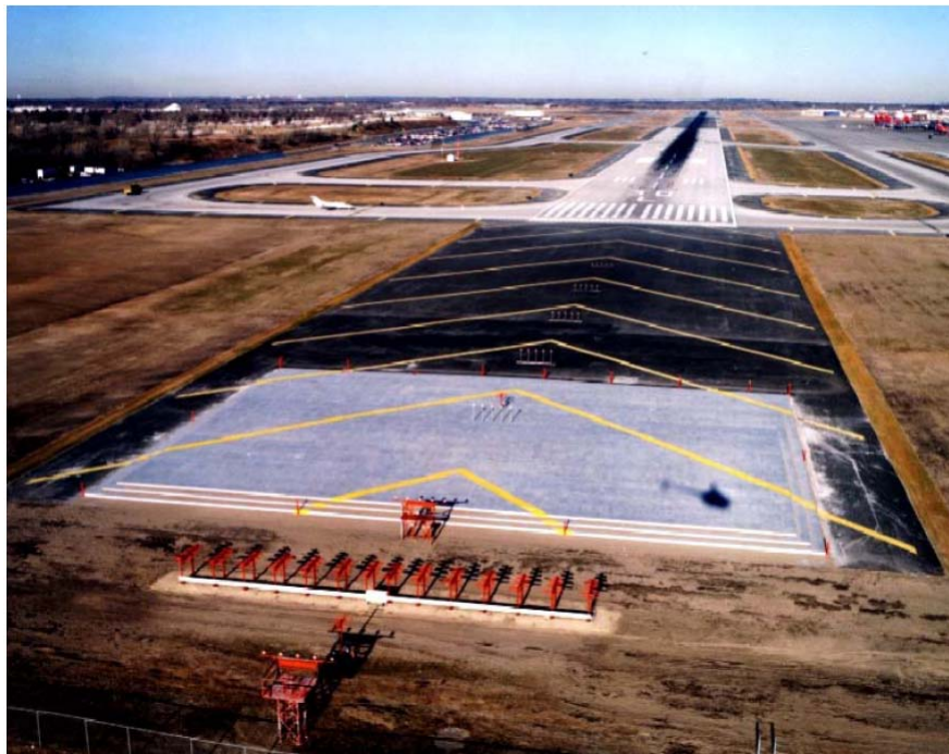
FIG AD 1.1-56 Engineered Materials Arresting System (EMAS)
