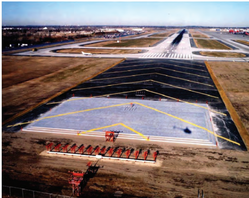
FIG AD 1.1-54 Engineered Materials Arresting System (EMAS)
