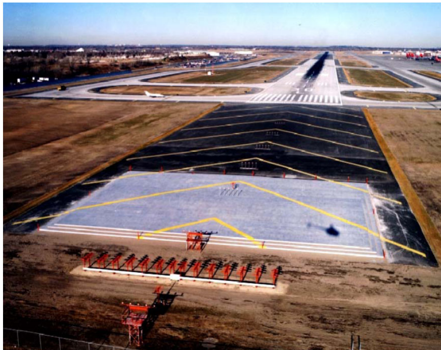
FIG AD 1.1-54 Engineered Materials Arresting System (EMAS)
