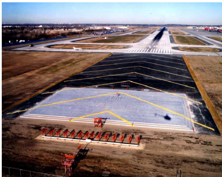
FIG AD 1.1-54 Engineered Materials Arresting System (EMAS)
