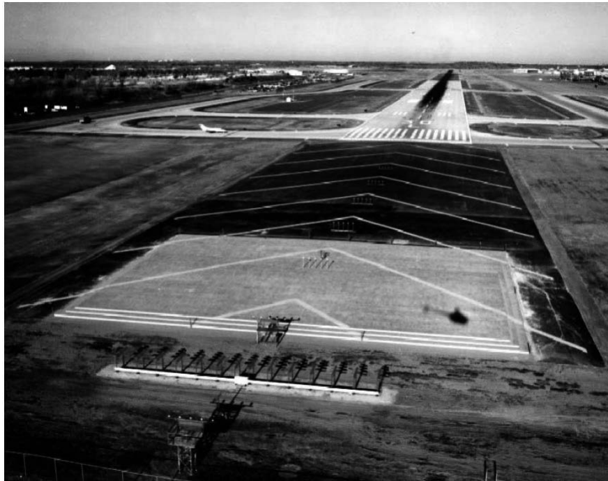
FIG AD 1.1-54 Engineered Materials Arresting System (EMAS)
