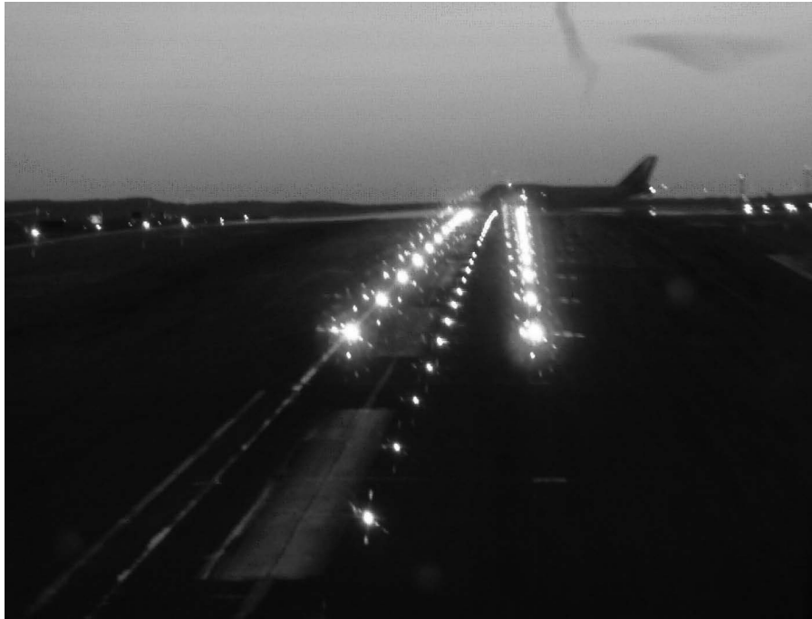
FIG AD 1.1-11 Takeoff Hold Lights
