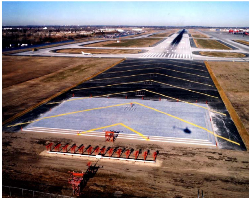
FIG AD 1.1-54 Engineered Materials Arresting System (EMAS)
