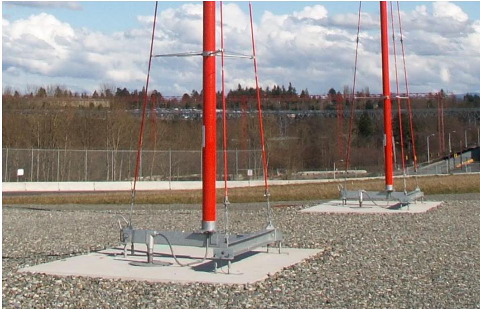
Standard Low Impact Resistant (LIR) structure installation with frangible bolts and flush gravel maintenance plot
