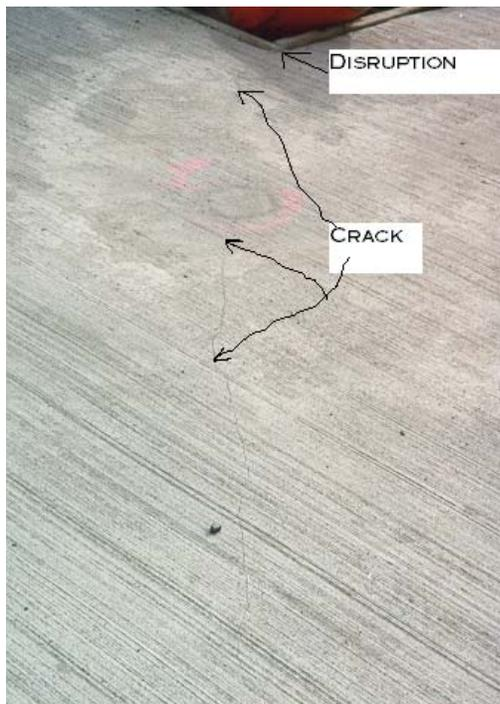
Photo 1 - Pavement Crack
