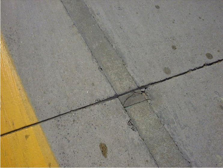
Photo 3 - Joint Spall at Electrical Duct
