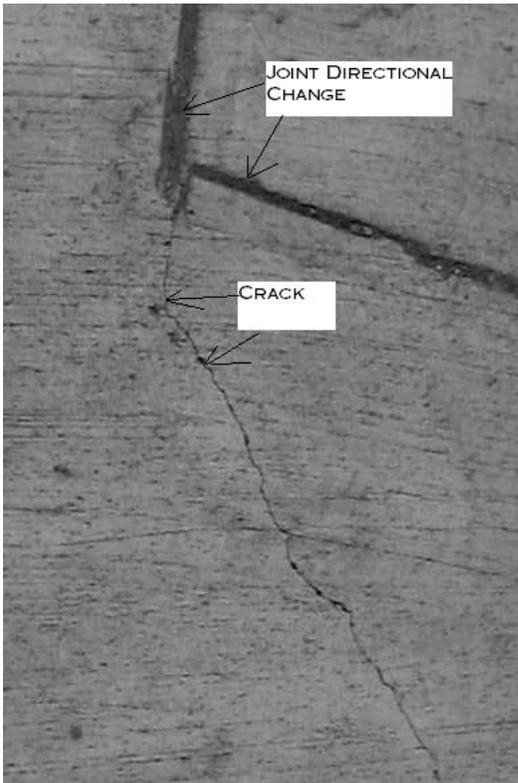
Photo 2 - Pavement Crack
