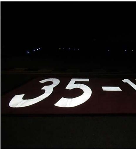
Type I glass beads must be used in the red background paint on surface painted holding position signs (SPHPS).
