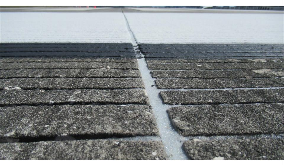
Excess glass beads, which are not properly removed, are considered Foreign Object Debris. This was found on an active runway during an FAA inspection.
