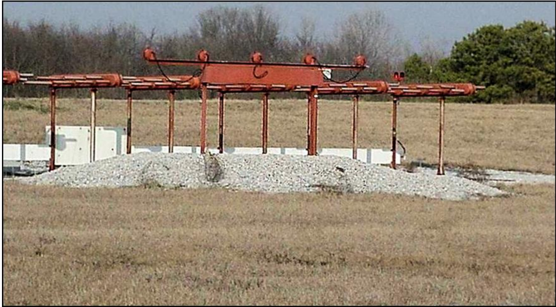
Excessive gravel fill creates a hazard
