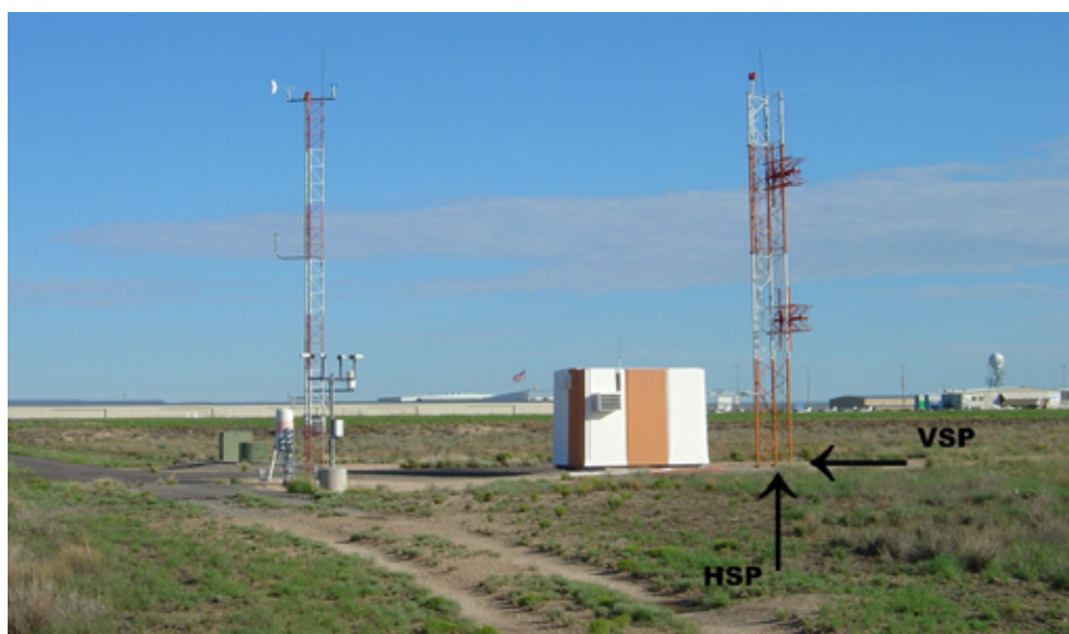
Figure C-6. Typical glideslope installation.
