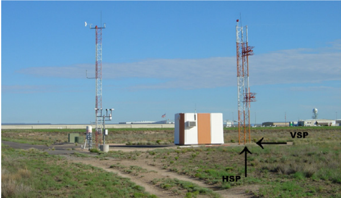
Figure C-6. Typical Glideslope Installation.
