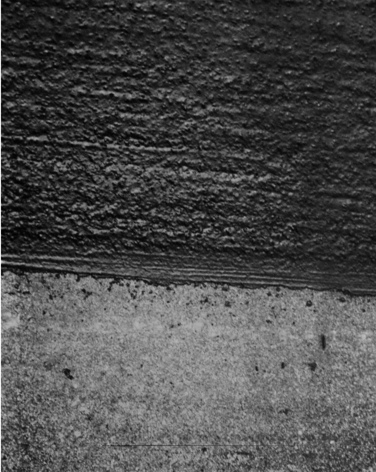
FIGURE 2-2. AGGREGATE SLURRY SEAL
