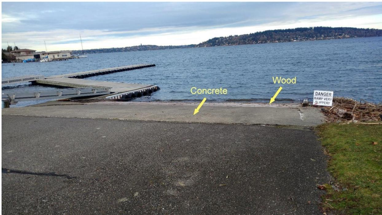
A typical ramp designed to accommodate seaplane floats is approximately 15 by 20 feet (5 m by 6 m) wide and extends into the water to allow seaplanes to be launched and retrieved easily. The ramp needs to be sized appropriately to accommodate the aircraft that will be using it. When determining the width and depth, take into account any
