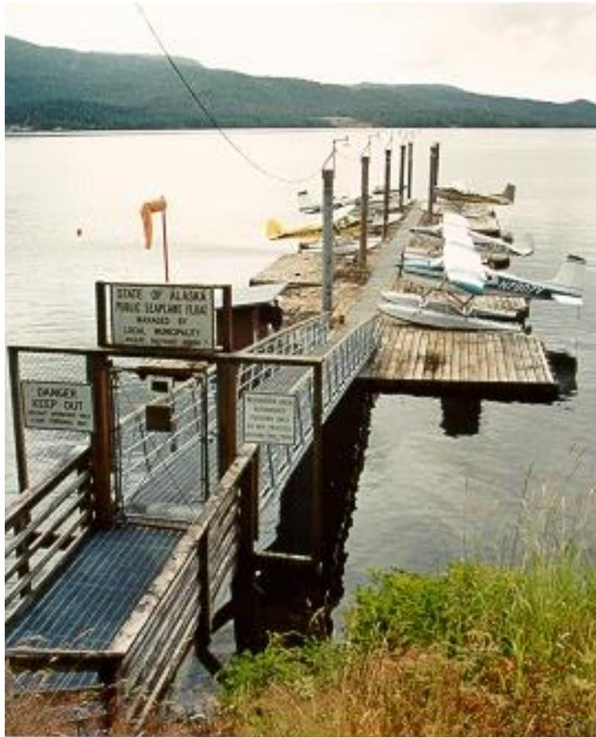
To permit movement, flexible interconnect systems should be used for attaching floats together or for attaching gangways. Typically hinge systems are used. Hinge systems may have removable pins to enable gangways to be disconnected for maintenance or reconfiguration, if needed. In the case of gangways affixed to the shore or to a fixed
