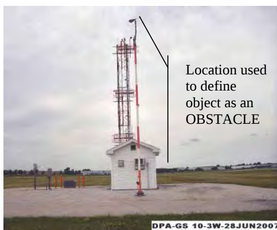
Figure 1-4. Illustrates the documentation of a glideslope antenna from different perspectives.
