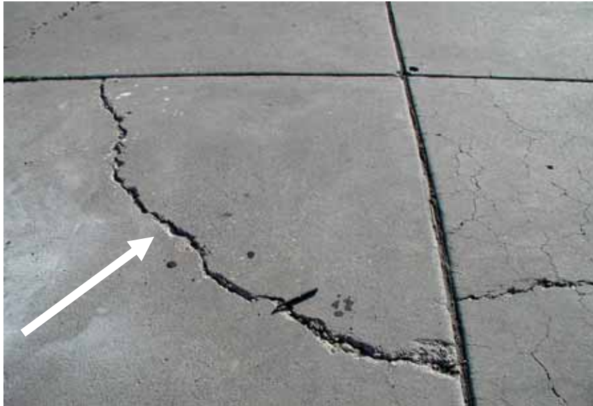
Figure 2-16. Corner break (→) in an airfield pavement.
