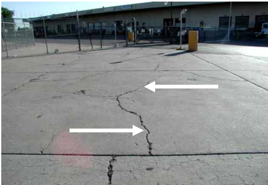
Figure 2-19. Longitudinal cracks (→) in an airfield pavement.
