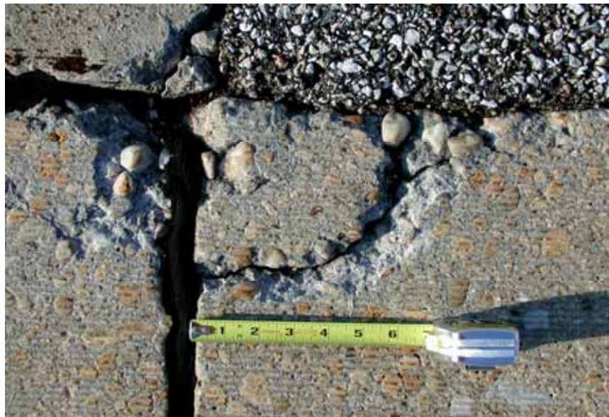
Figure 2-17. Corner spall in another airfield pavement.
