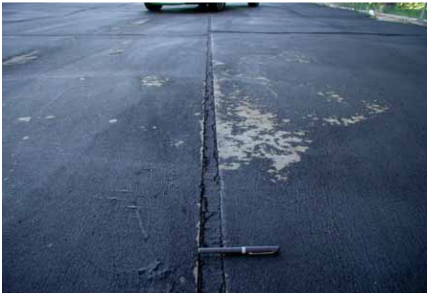
Figure 2-14. Heaving of a slab relative to another
