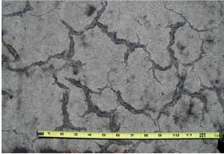
Figure 2-9. Gel exudation through cracks.
