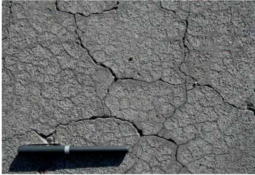
Figure 2-5. Severe map cracking.
