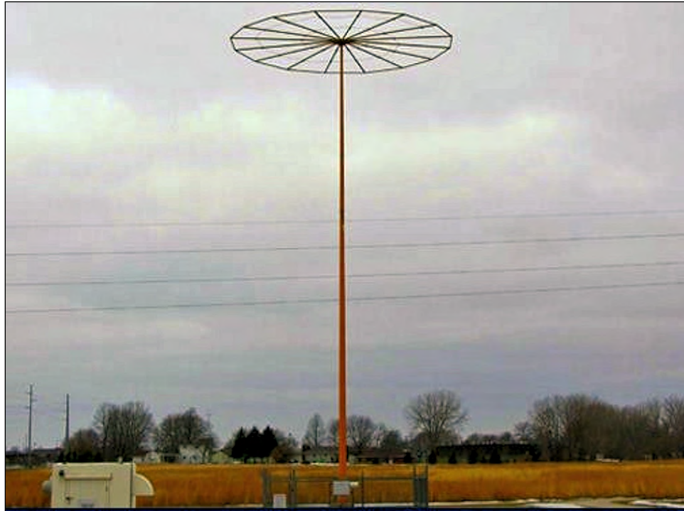
Figure 6-23. Non-Directional Beacon (NDB) Facility
