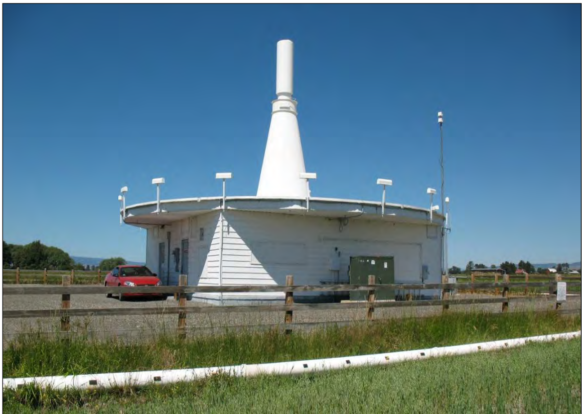
Figure 6-21. Enroute VHF Omnidirectional Range (VOR) Facility
