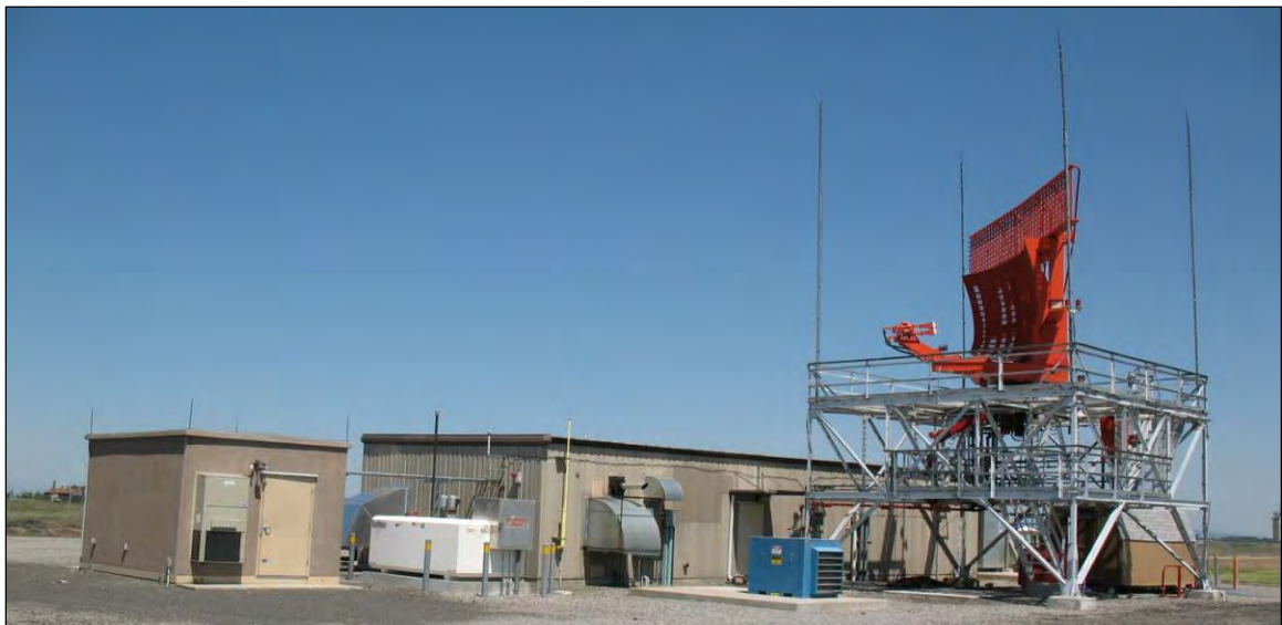
Figure 6-6. Airport Surveillance Radar (ASR) Steel Tower (17 feet (5.2 m) high)
