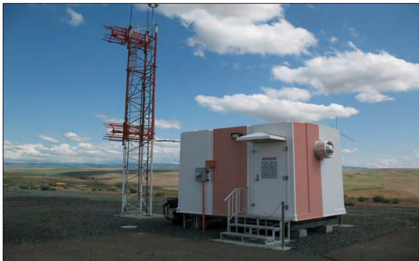
Figure 6-18. GS Antenna and Equipment Shelter
