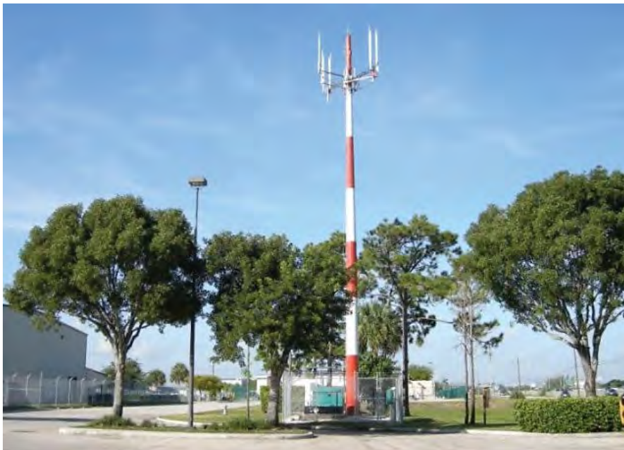
Figure 6-29. Automated Dependent Surveillance Broadcast (ADS-B) Ground Station
