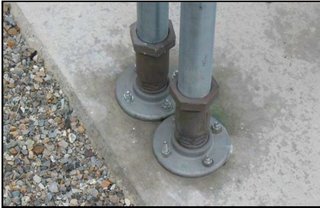
Figure 6-4. Two Frangible Connections
