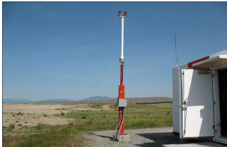
Figure 6-19. Distance Measuring Equipment (DME) Antenna
