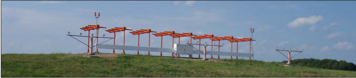
Figure 6-16. LOC 8-Antenna Array
