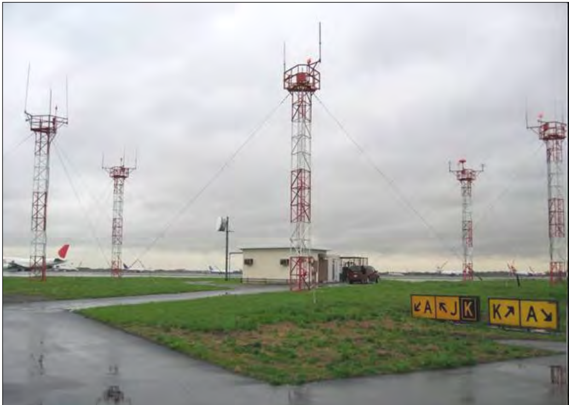
Figure 6-5. Remote Transmitter/Receiver (RTR) Communication Facility
