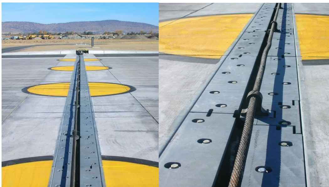
Figure A-20. Plan View of Typical BAK-12/14 (or Type H) Installation
