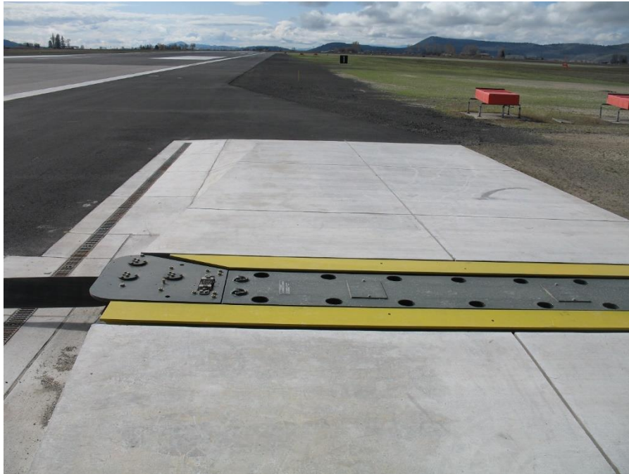
Figure A-13. Fairlead Beam and Ramp
