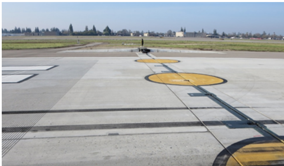
Figure A-18. BAK-14 with Fairlead Beams and Pit—Note no grooving 10 feet within cable
