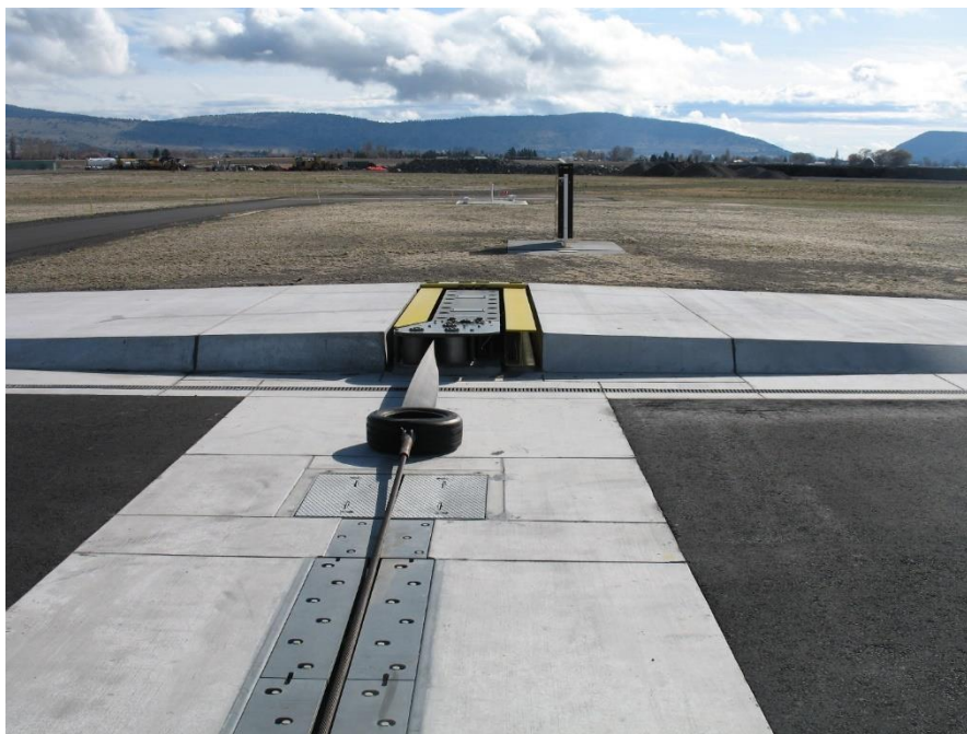
Figure A-12. Type H System with Fairlead Beam and Ramp and BAK-12 Pit in Background
