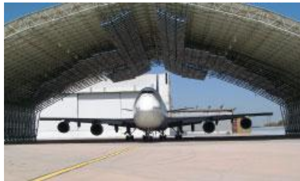
Figure 5-1. Infra-red deicing facility at John F. Kennedy International Airports with the Boeing 747-200.
