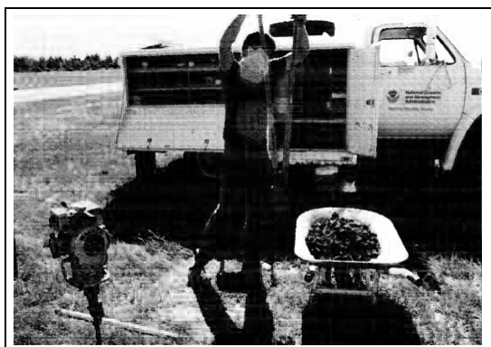
Figure 8.18. Digging the 43" deep hole; 12"- 14" diameter for the top 22" in depth, and 3"- 6" diameter for the bottom 21" (Note, Dirt removed with a wheelbarrow)
