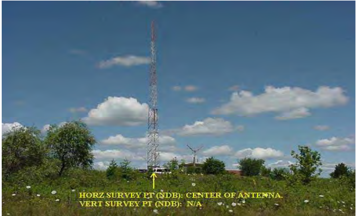
Figure 8.10. Is a NAVAID photo with the horizontal and vertical survey points identified.
