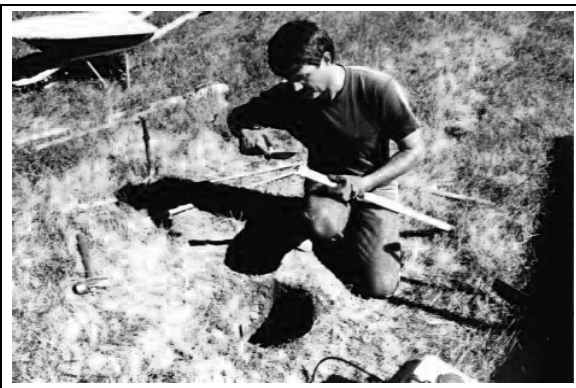
Figure 8.23. Preparing one-inch PVC grease filled "finned" sleeve.
