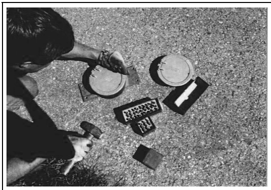
Figure 8.17. Stamp the station designation on the collar of the logo cap.
