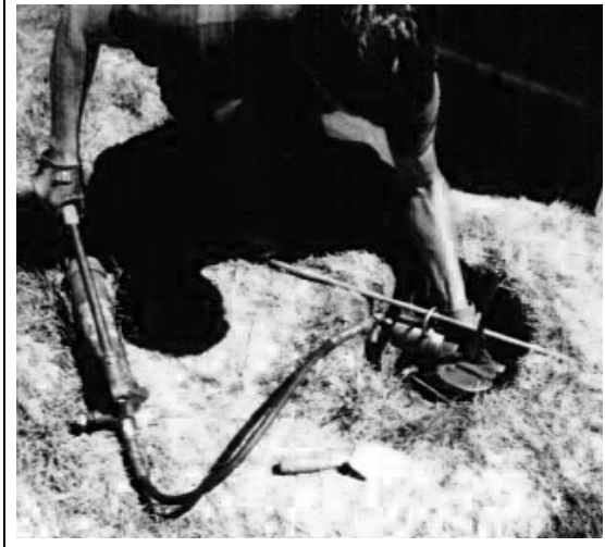
Figure 8.21. Cutting off the top of the stainless steel rod using a hydraulic cutter approximately 3 inches below the surface.
