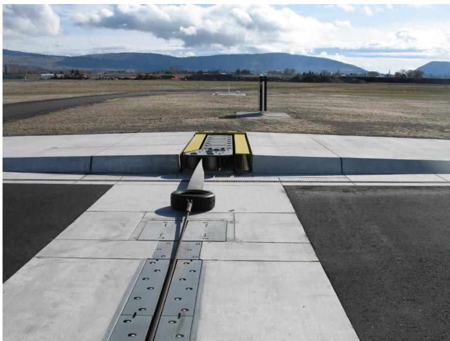
Figure A-9. Type H System with Fairlead Beam and Ramp and BAK-12 Pit in Background
