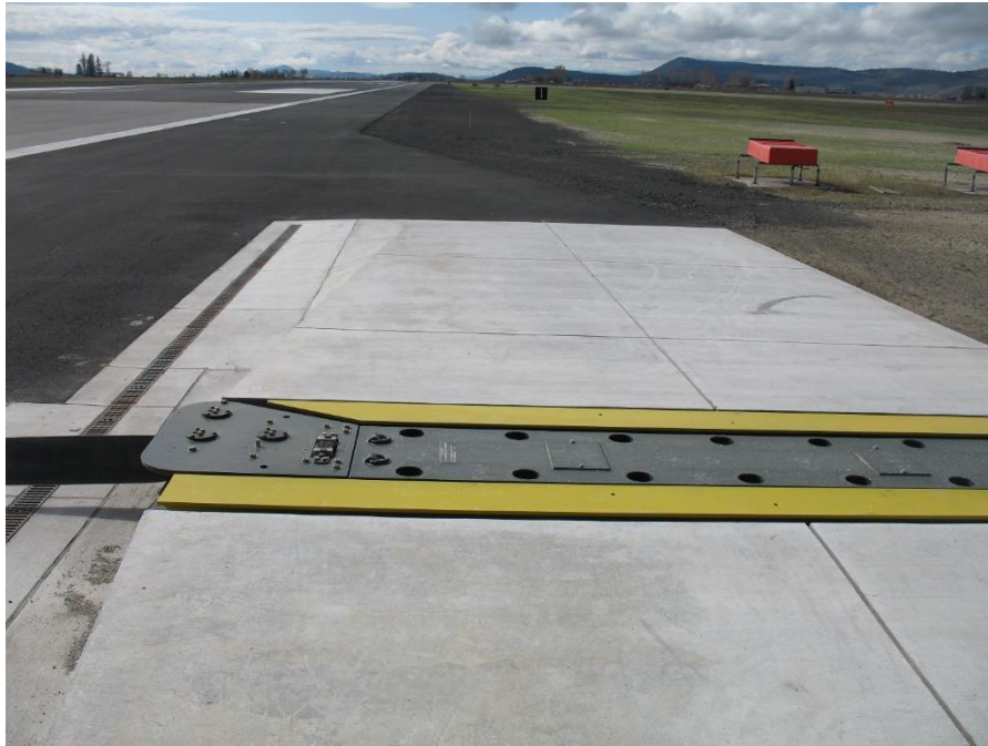
Figure A-10. Fairlead Beam and Ramp
