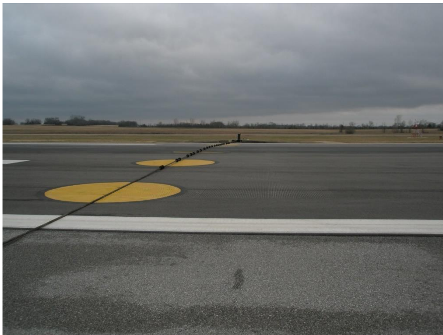
Figure A-15. BAK-14 with Fairlead Beams and Pits—Note no grooving 10 feet within cable
