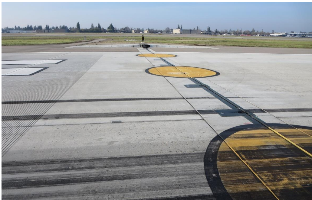
Figure A-15. BAK-14 with Fairlead Beams and Pits—Note no grooving 10 feet within cable
