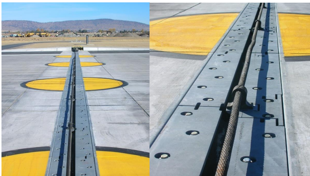
Figure A-17. Plan View of Typical BAK-12/14 (or Type H) Installation
