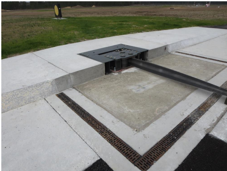
Figure A-13. Figure A2-5. Edge Sheave and Ramp (Side View)
