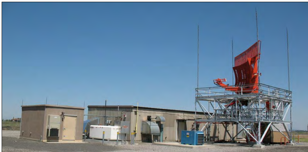
Figure 6-6. Airport Surveillance Radar (ASR) Steel Tower (17 feet [5 m] high)
