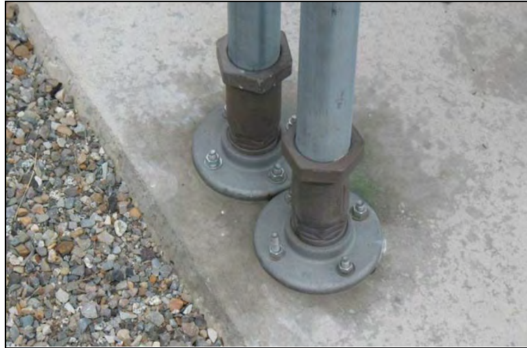
Figure 6-4. Two Frangible Connections
