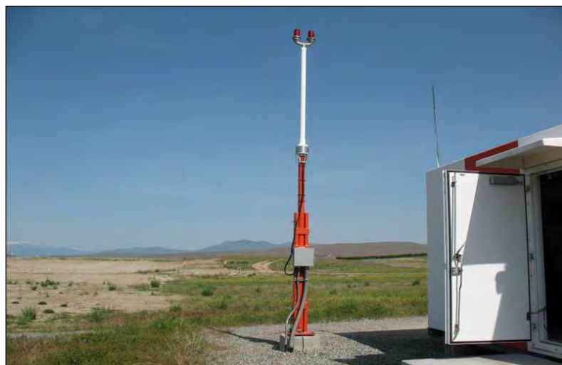
Figure 6-20. Distance Measuring Equipment (DME) Antenna
