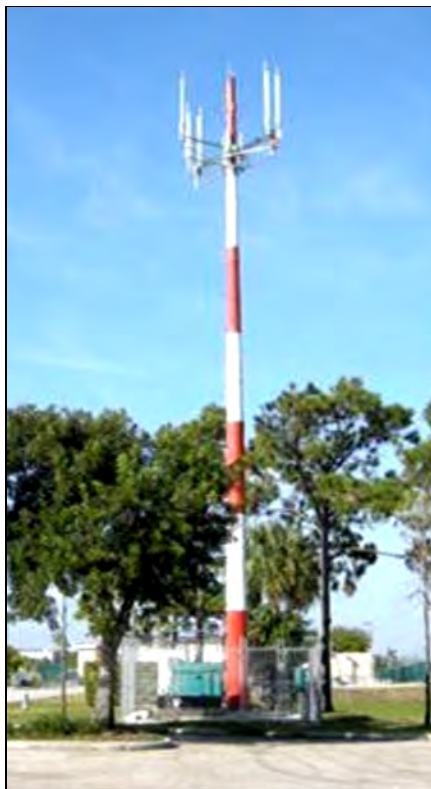
Figure 6-29. Automated Dependent Surveillance Broadcast (ADS-B) Ground Station
