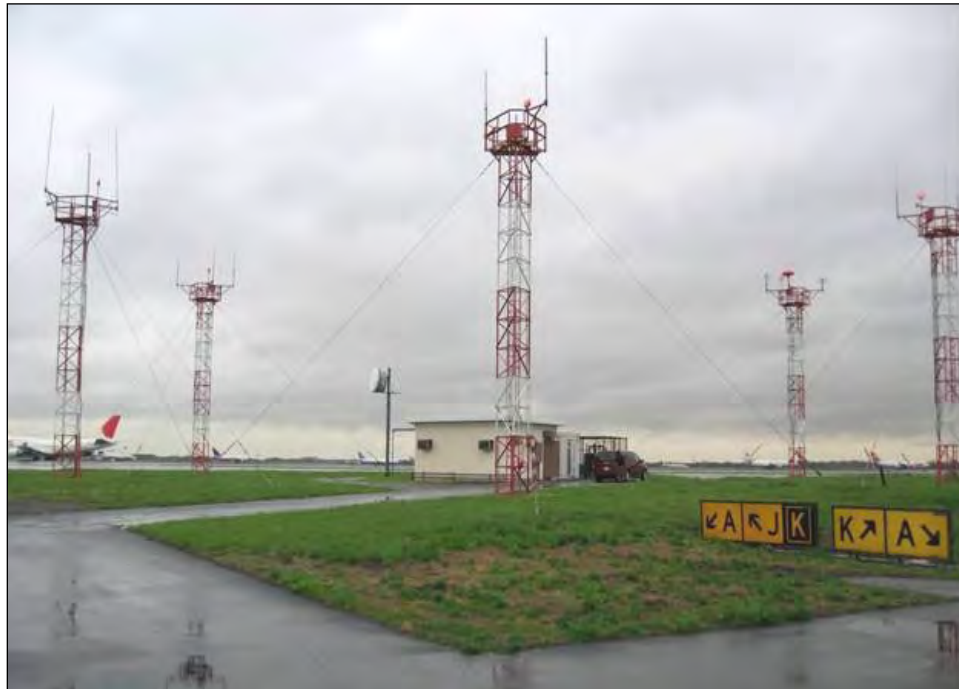
Figure 6-5. Remote Transmitter/Receiver (RTR) Communication Facility
