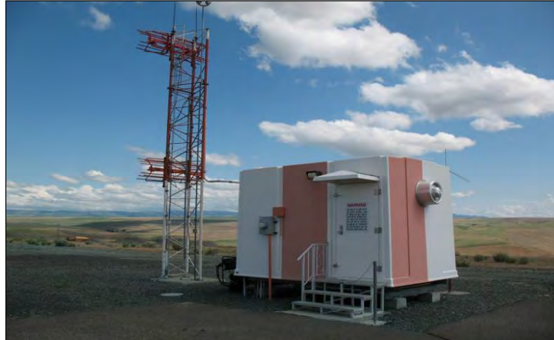
Figure 6-19. GS Antenna and Equipment Shelter
