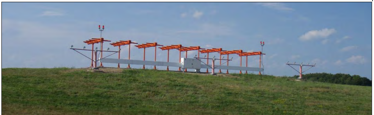
Figure 6-17. LOC 8-Antenna Array
