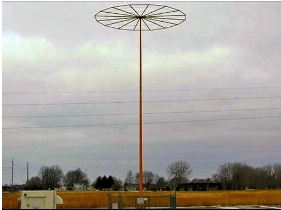
Figure 6-24. Non-Directional Beacon (NDB) Facility
