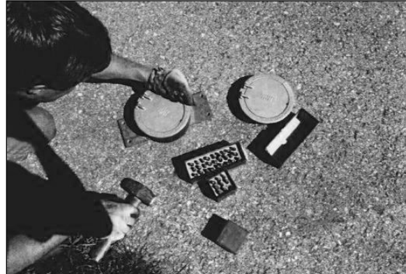
Figure 7-11. Stamp the station designation on the collar of the logo cap.
