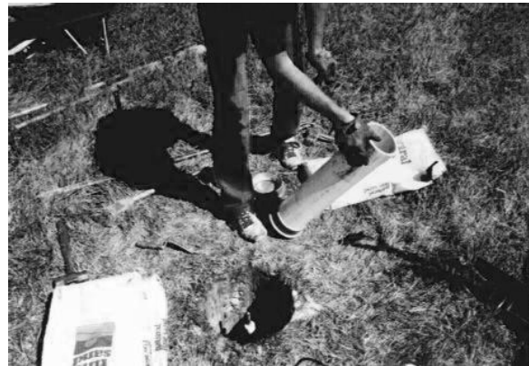
Figure 7-19. Preparing to place 5 or 6 inch PVC pipe over and above the centered grease sleeve and stainless steel rod.
