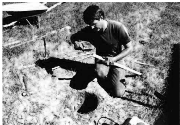
Figure 7-17. Preparing one-inch PVC grease filled “finned” sleeve.
