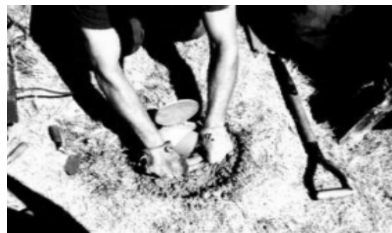
Figure 7-22. Shaking the PVC pipe to settle concrete and fill any voids.
