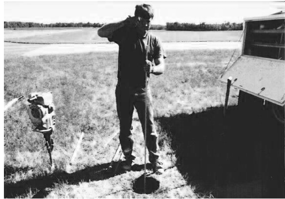
Figure 7-13. Starting the stainless steel rod with a hammer.
