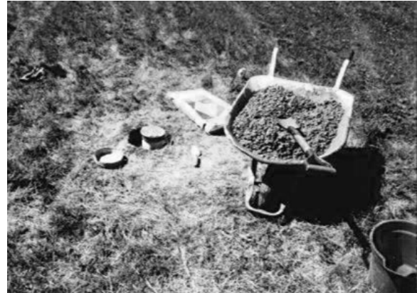
Figure 7-20. Mixing concrete for use in completing the monument.
