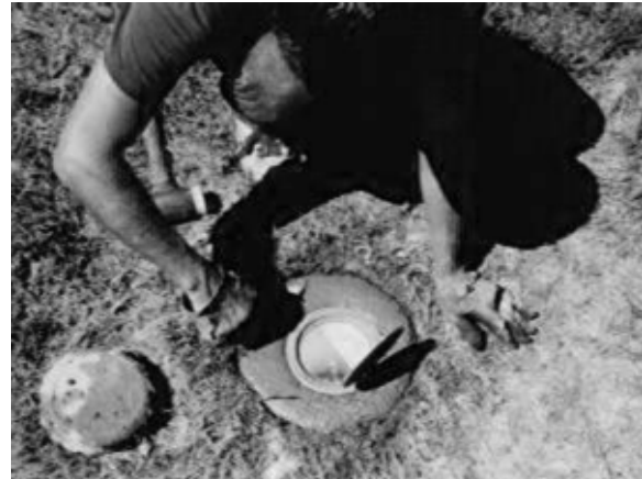
Figure 7-23. Trowel the top of the concrete until there is a smooth finished surface.
