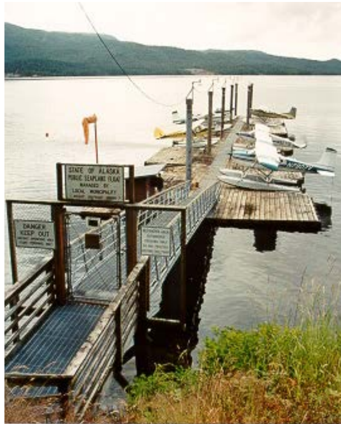
Figure 4-9. Example of a Gangway in Alaska
