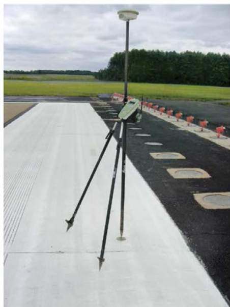
Incorrectly placed survey equipment
