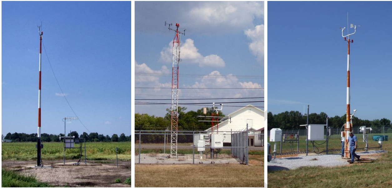
Figure 2-11. SAWS, AWOS and ASOS Station Installations.
