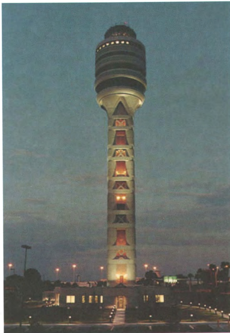
Orlando Airport Traffic Control Tower
