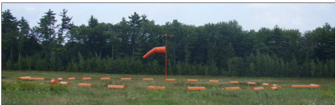
Figure 6-32. Segmented circle and wind cone
