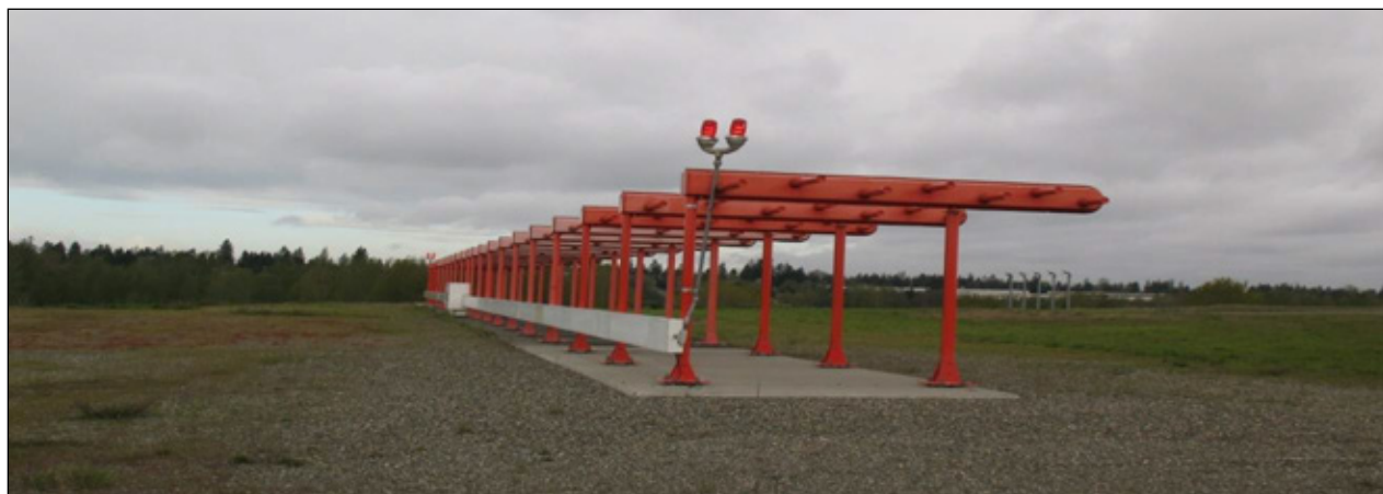
Figure 6-22. LOC 14-antenna array
