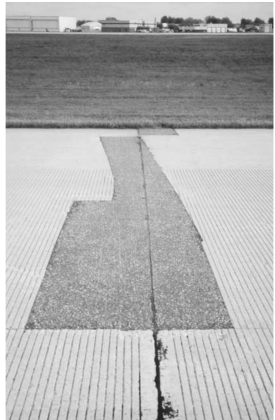
▲ Full depth joint repair. Very good condition.
