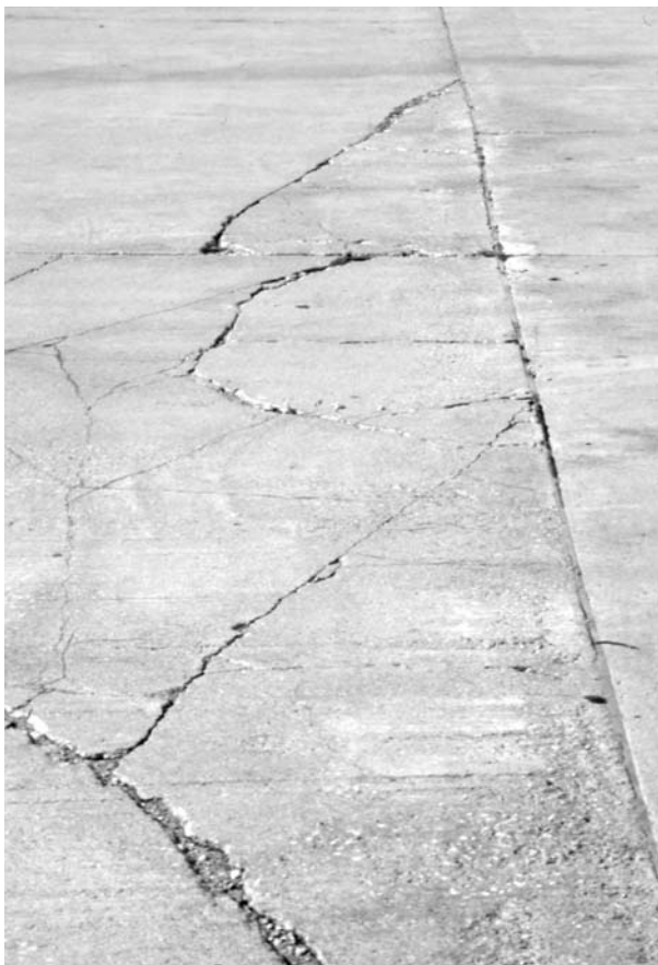
▲ Multiple slab cracks, spalling and shattered slabs.
