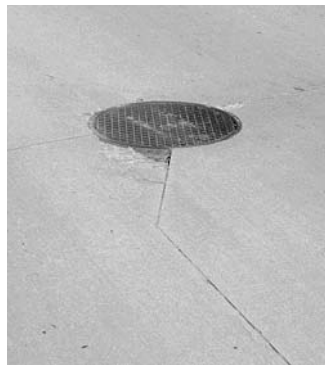
▲ Isolated spall at manhole.
