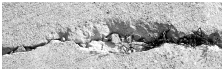
◀ Spalling along a joint.
