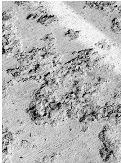
◀ Severe scaling. Some larger aggregate is loose.
