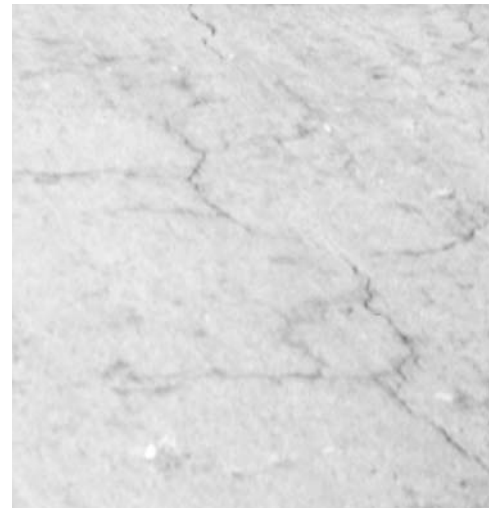
▲ Map cracking, but pavement is sound.
