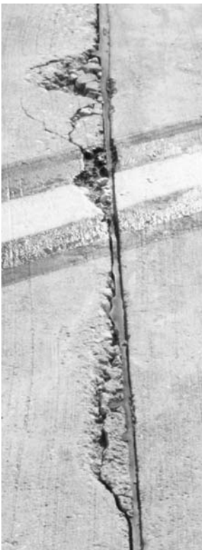
◀ Spalling along a joint.
