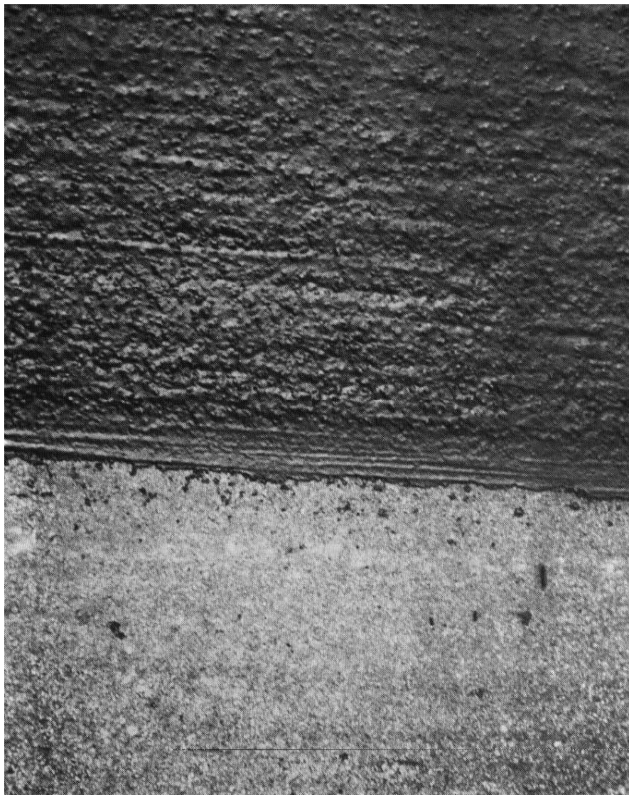
Figure 2-1. AGGREGATE SLURRY SEAL
