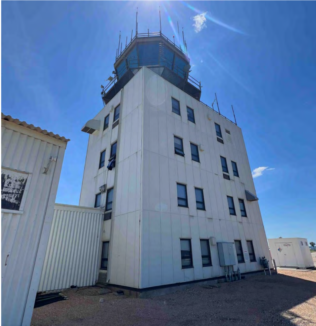
Figure 1-2. Photo of Existing Non-standard Design FCM Tower
